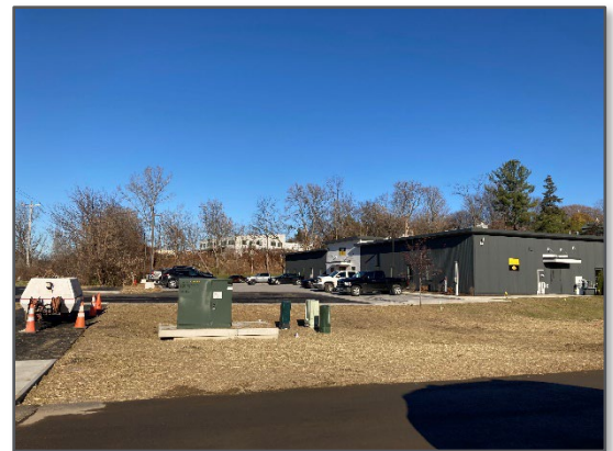
The new American Railway Dispatch Center at the Fonda brownfield cleanup site. [Photo: VEPC staff.]
