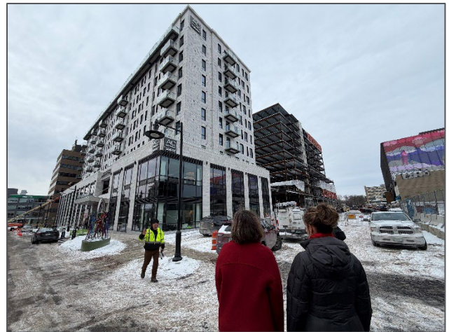
City Place under construction. [Photo: VEPC staff.]
