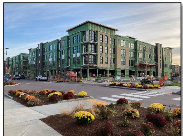
Catamount Run buildings under construction. [Photo: VEPC staff]
