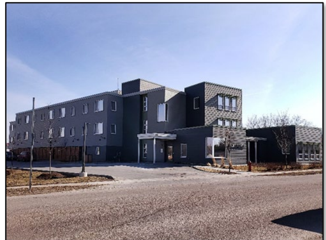
Elm Place offers affordable senior housing in Milton's Town Core. It was constructed in 2017 and is Vermont's first multifamily "passive house" building. [Photo: Town of Milton.]
