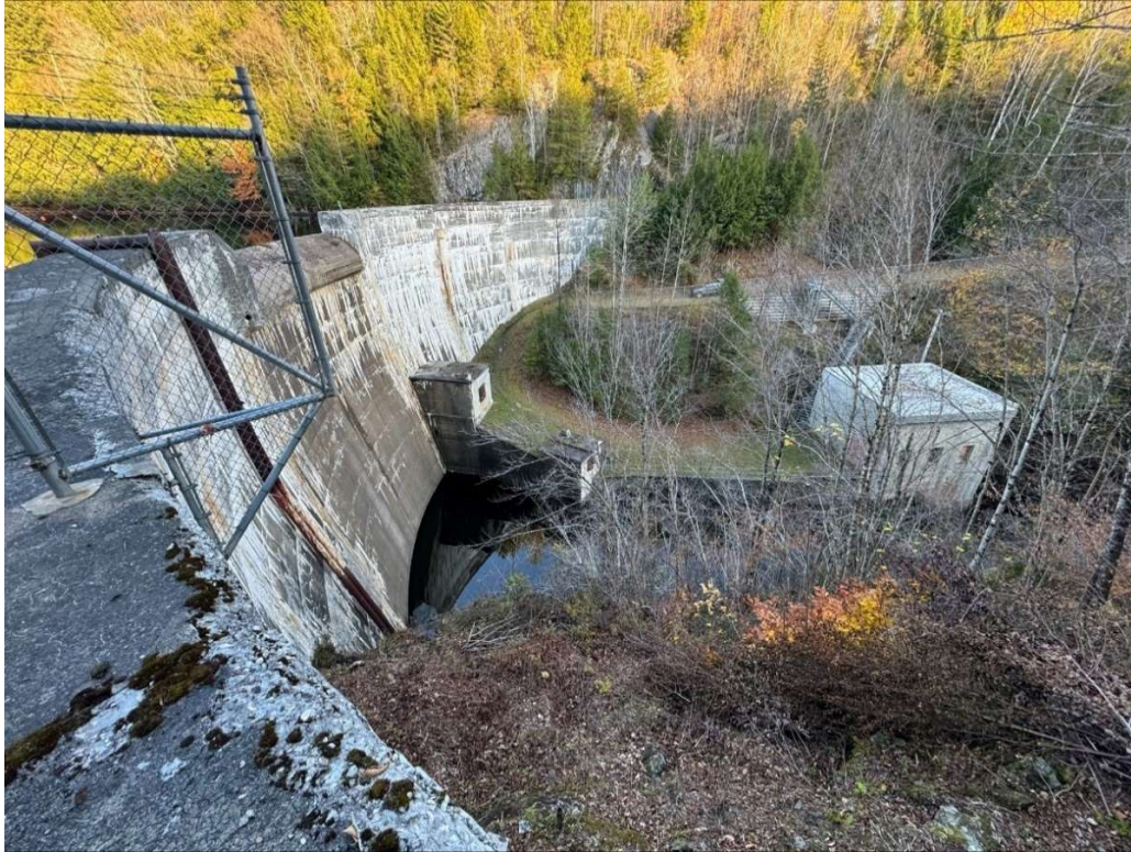
Figure 5: Downstream face of concrete arch dam and valve/gate buildings (9-18-2024).
