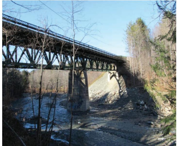
**BETHEL.** The Bethel VT Route 12 Bridge 38 project replaces the existing four-span steel deck trusses. Traffic is currently being maintained on the existing bridge while the new bridge is constructed upstream of the existing structure. When the project was contracted, a flood came through and stabilization had to take place for the road to remain open.
