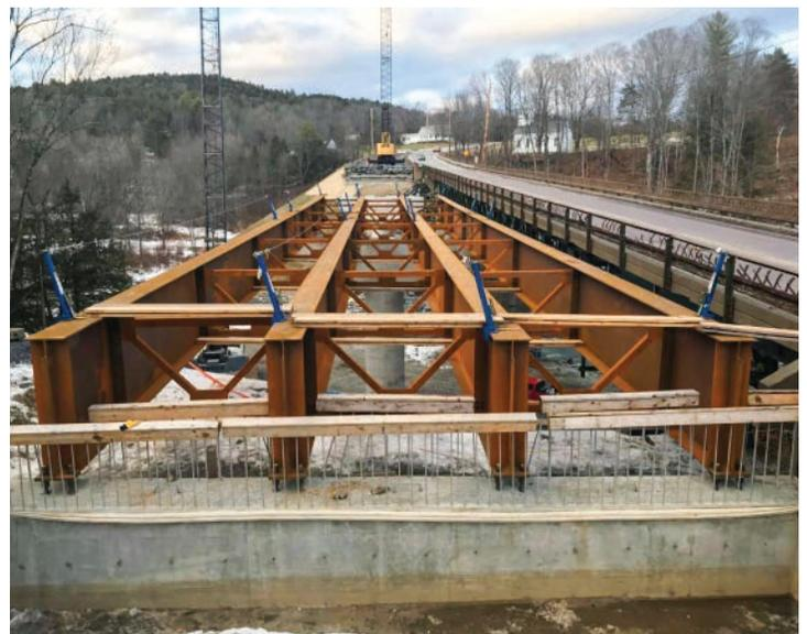
**BETHEL.** The new three-span bridge has a weathering steel plate girder superstructure. The new bridge is 364 feet long including two approach spans of 110 feet and a center span of 144 feet. An ornamental steel lattice treatment similar to that on the existing bridge will be attached to the outside of the standard two-rail box beam for aesthetic purposes.
