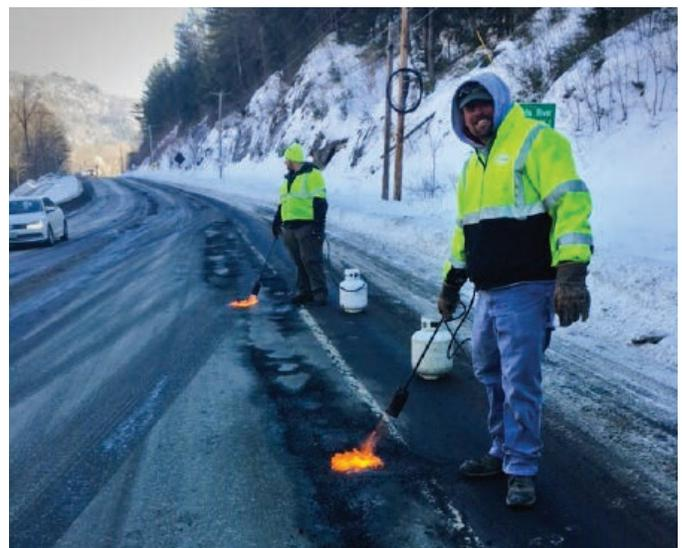
**GROTON.** Pothole patching can be an effective temporary fix but often requires a little heat in colder months to help the material stick to the road surface.
