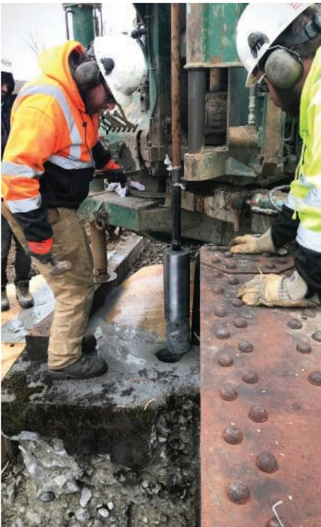
**COVENTRY.** All VTrans construction projects require proper planning and usually bring together diverse parts of the agency. An upcoming rail project gathered Rail, Geological, and Materials crews to collect core samples for close inspection.
