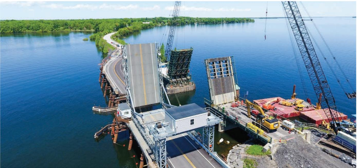
**NORTH HERO - GRAND ISLE.** Multi-year construction of the North Hero/Grand Isle drawbridge along US-2 continued throughout the year. 2019 saw the completion of the temporary bridge and the demolition of the old bridge decks. The new permanent drawbridge will be built in the footprint of the historic structure.
