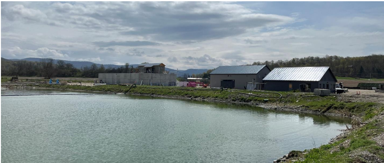
Figure 1. Hinesburg Vermont Wastewater Treatment Facility
