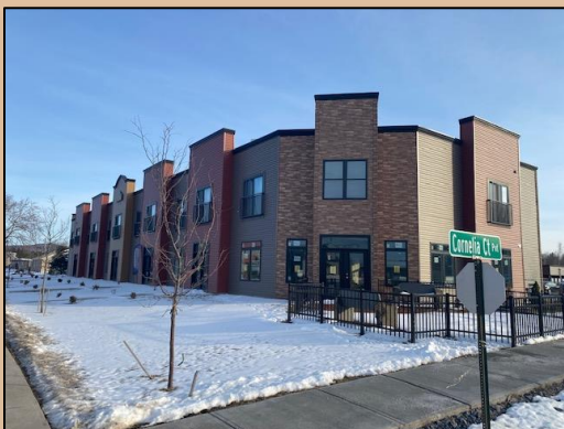
Completed Cornelia Court multiuse building which includes apartments, townhouses and commercial space.
