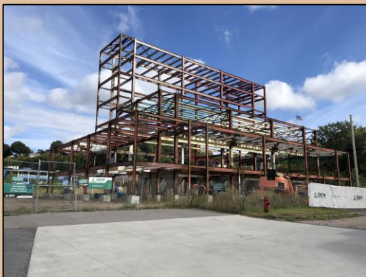
Partial demolition and site stabilization of the Moran Plant.
