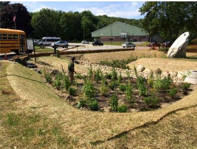
Figure 23. Stormwater treatment practice installed by Friends of the Mad River at Harwood Union Middle and High School; structure serves additional purpose as outdoor classroom to educate students on green stormwater infrastructure
