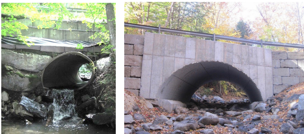
Figure 21. Before (left) and after (right) replacement of stream culvert at Hayes Road, Duxbury, completed by Friends of the Winooski River
