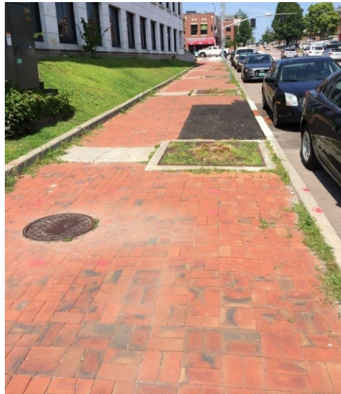
Figure 22. Before (left) and after (right) installation of a pervious sidewalk in downtown Burlington, completed by the City of Burlington
