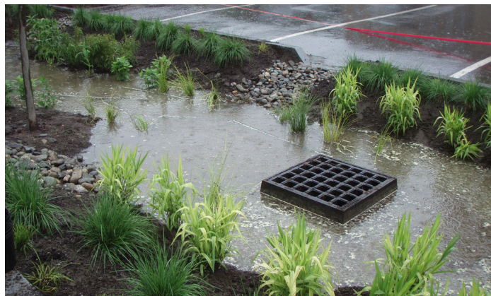
Bioretention basin infiltrating stormwater runoff
