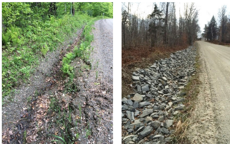
Figure 20. Before (left) and after (right) installation of a stone-lined ditch along Fayston Road, Fayston, completed by Friends of the Mad River
