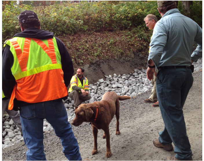
VTrans and DEC staff visiting a rock-lined and planted ditch, during a site visit
