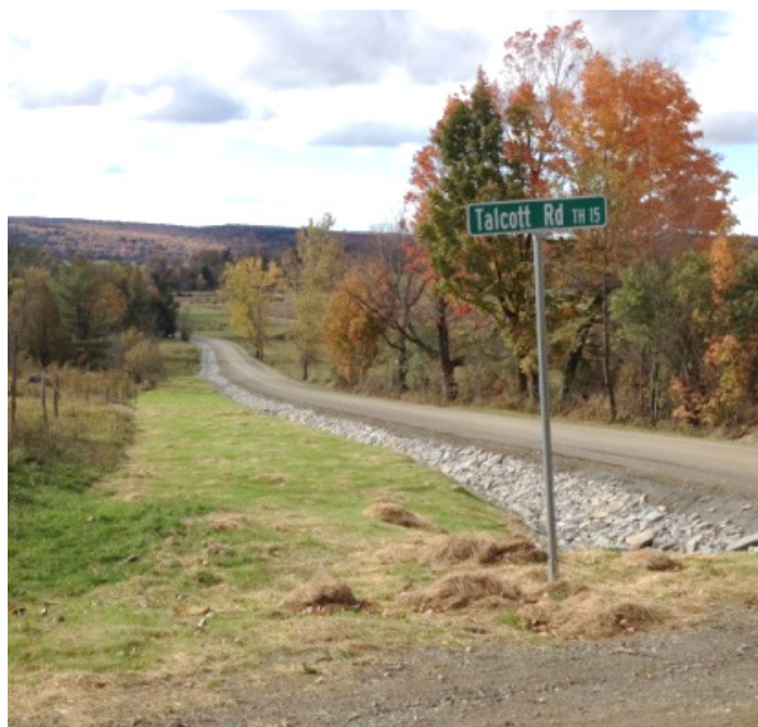
Stone-lined ditch project on Talcott Road, Fairfield, reducing road erosion
