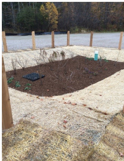
Figure 23. Before (left) and after (right) installation of a bioretention stormwater treatment structure installed at Lake Iroquois public beach parking lot, completed by the Lake Iroquois Recreation District
