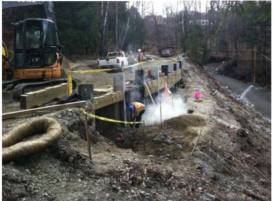
FIGURE 36 RAIL REPAIR IN VERMONT
