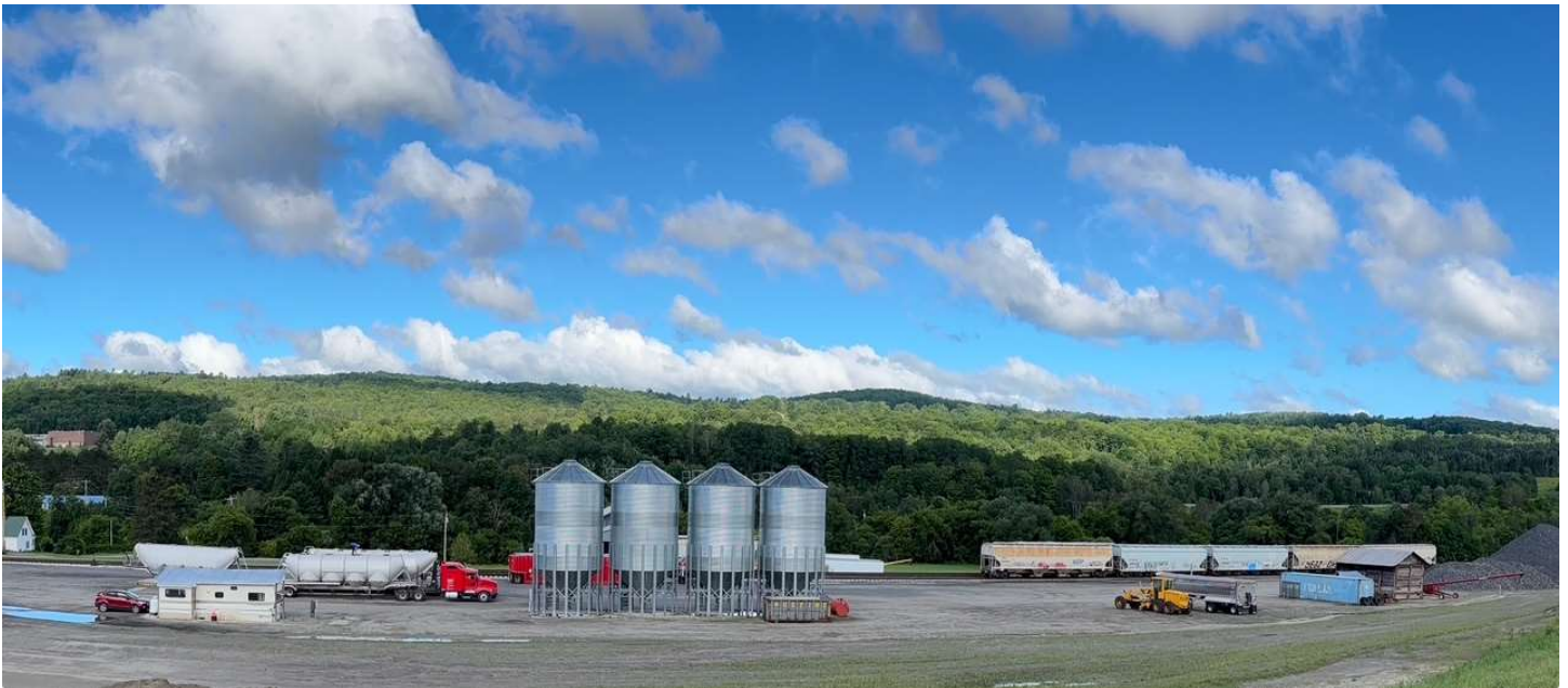
FIGURE 34 BARTON TRANSLOAD FACILITY
