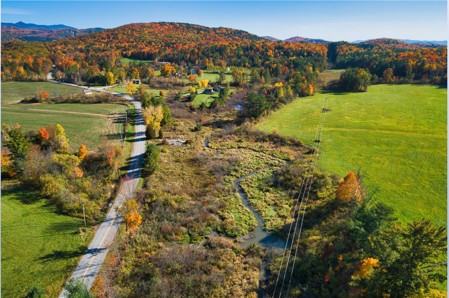
Wainwright Dam Removal and Wetland Restoration, FluidStateConsulting
