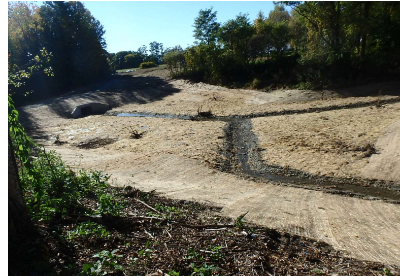
UVM Lower Dam Removal, South Burlington
