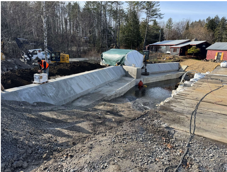
Curtis Pond Dam Rehabilitation, Calais
