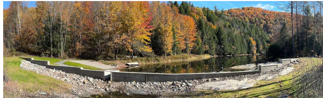
Gillett Pond Dam Replacement, Richmond
