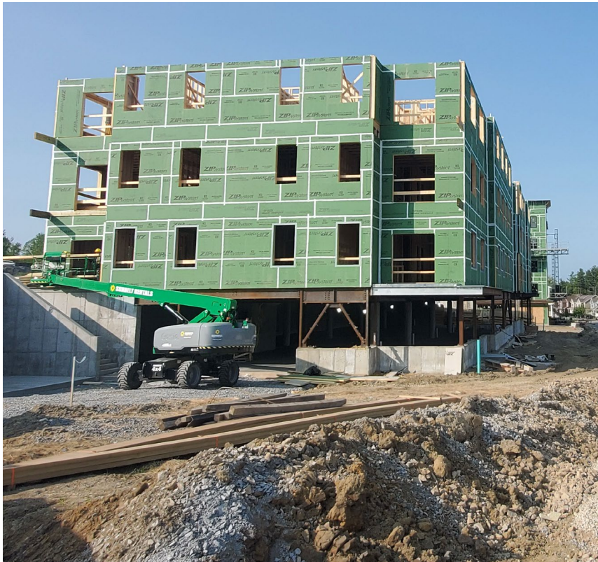
O'Brien Farms in South Burlington, under construction
