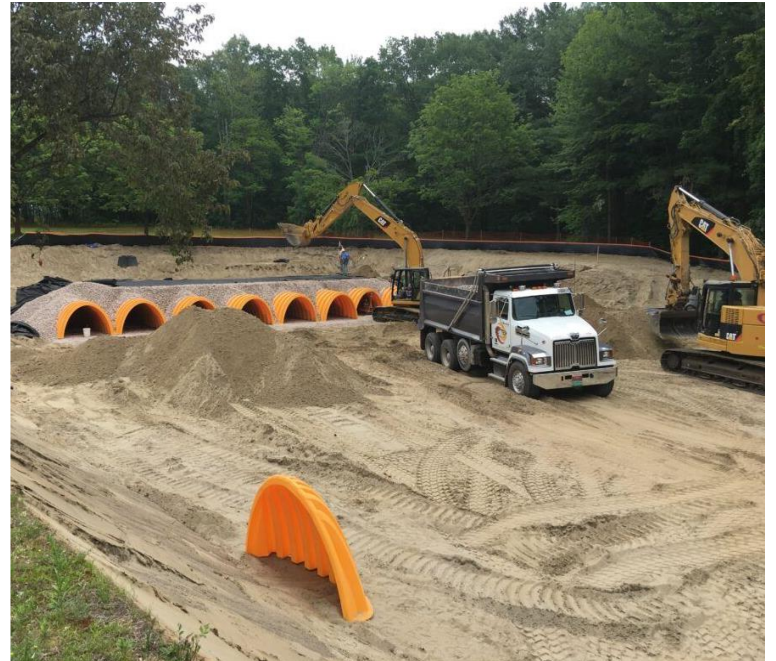
Picard Circle, South Burlington:: Underground stormwater infiltration system in construction
