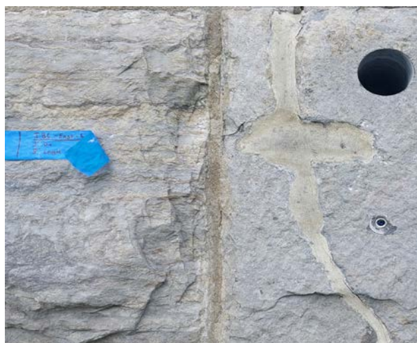
Image 74. Caulk repair and current core hole
