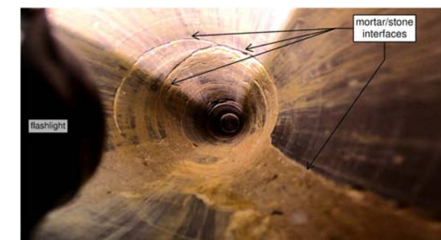
Image 22. Between interior and exterior face wythes, CORE-NORTH. Atkinson-Noland & Associates
