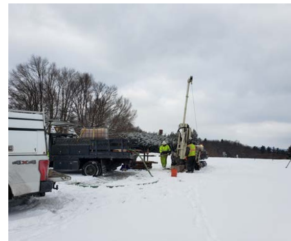
Image 53. Geotech Drilling. Stevens & Associates 01.17.2024
