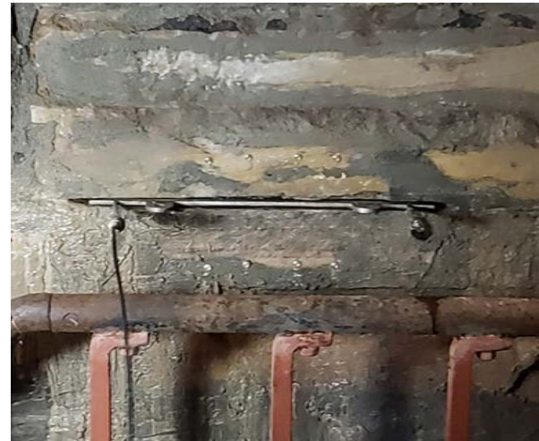
Image 12. Flat Jack Test. Stevens & Associates 07.17.2023
