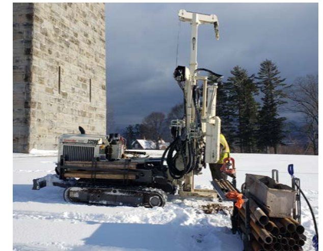
Image 55. Geotech Drilling. Stevens & Associates 01.17.2024
