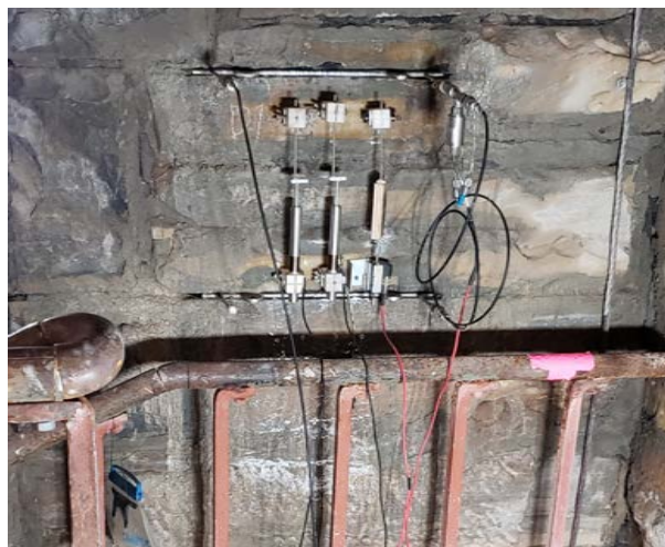
Image 13. Flat Jack Test. Stevens & Associates 07.17.2023
