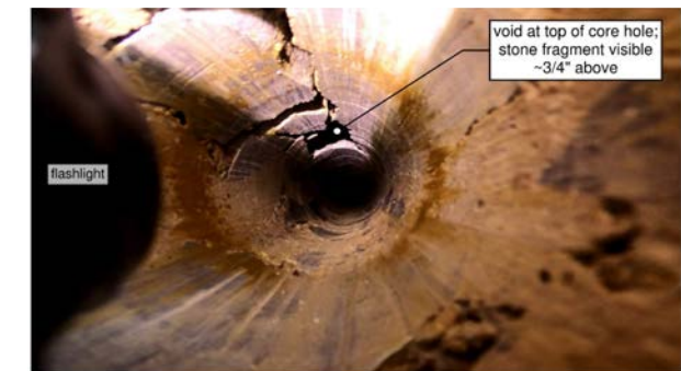
Image 21. Between interior and exterior face wythes, CORE-NORTH. Atkinson-Noland & Associates
