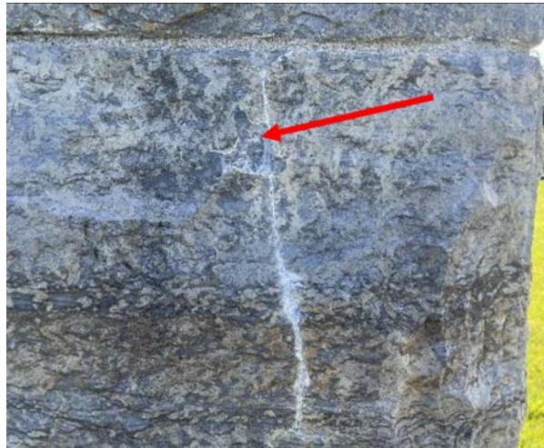
Image 51. Shallow spall. Jablonski
