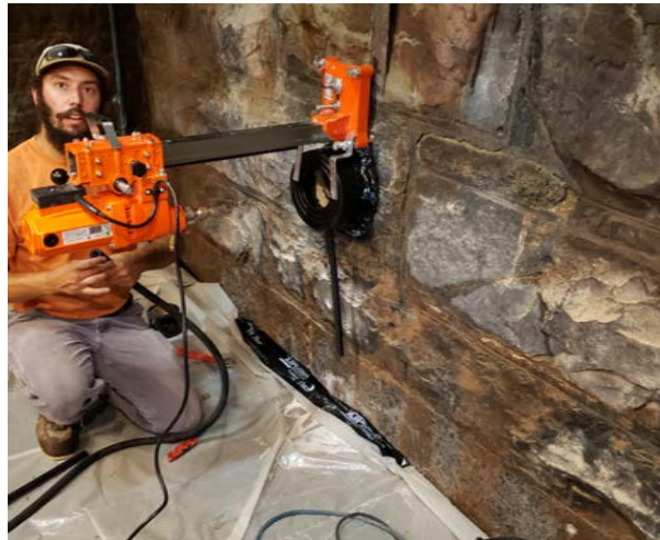
Image 15. Goodman Jack Test. Stevens & Associates 07.17.2023
