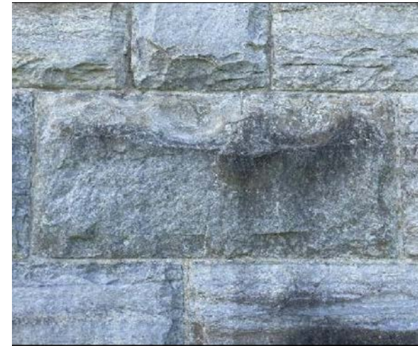
Image 33. Typical exterior condition. Jablonski
