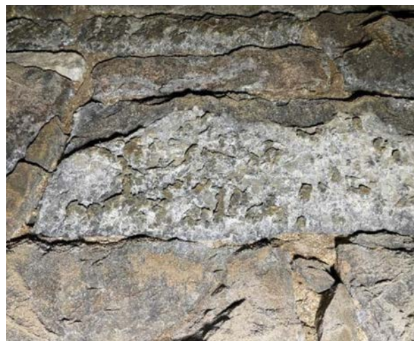
Image 34. Uneven surface texture of dark gray stone unit. Jablonski
