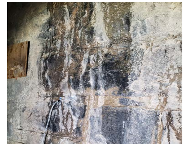
Image 56. Geotech Drilling. Stevens & Associates 01.17.2024
