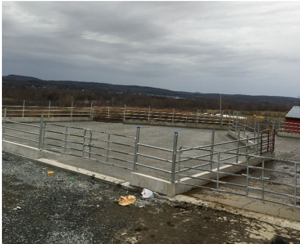
Before (top) and after (bottom) installation of a Heavy Use Area Protection practice to address runoff and erosion risks in the Missisquoi watershed.
