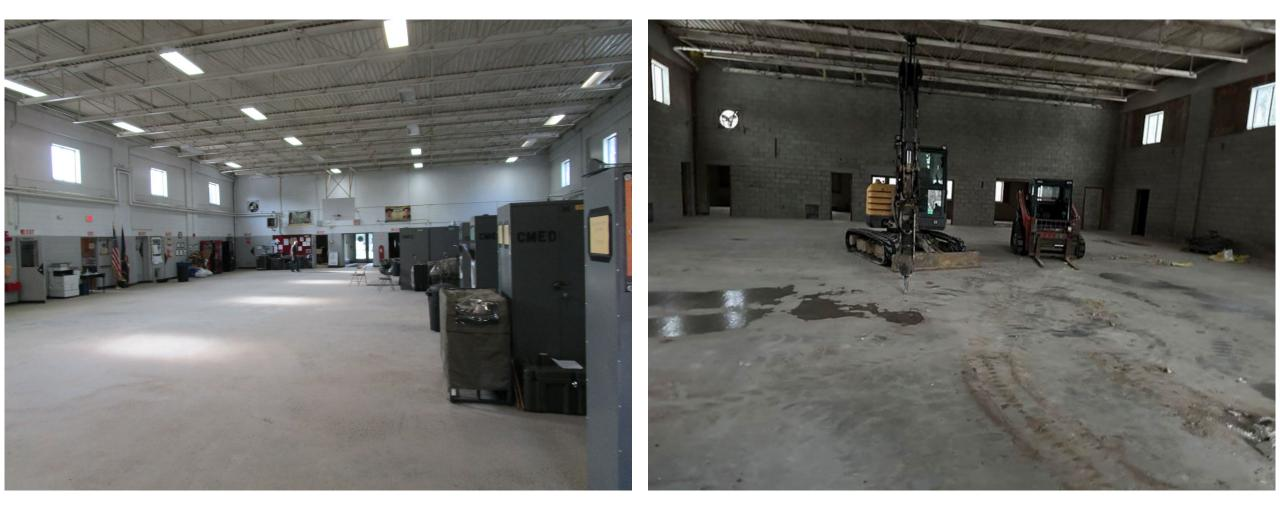
Demolition is currently underway at Winooski. Shown above is the drill hall before and after sandblasting surfaces to remove all hazardous materials prior to the building being demolished. Estimated completion spring 2025.
