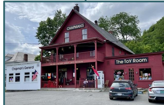
Chapman's General Recently invested $1.3m into business expansion and workforce housing. Currently under construction.
