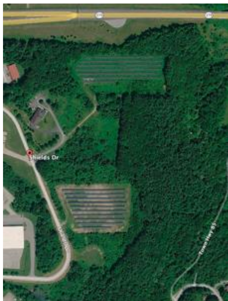
Furnace Brook Solar LLC Solar 1.65 MW
