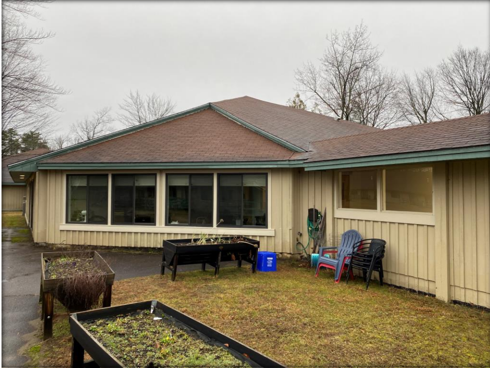
Whitcomb Woods Constructed 1980 by private owner 65 apartments with Section 8 Rental Subsidy
