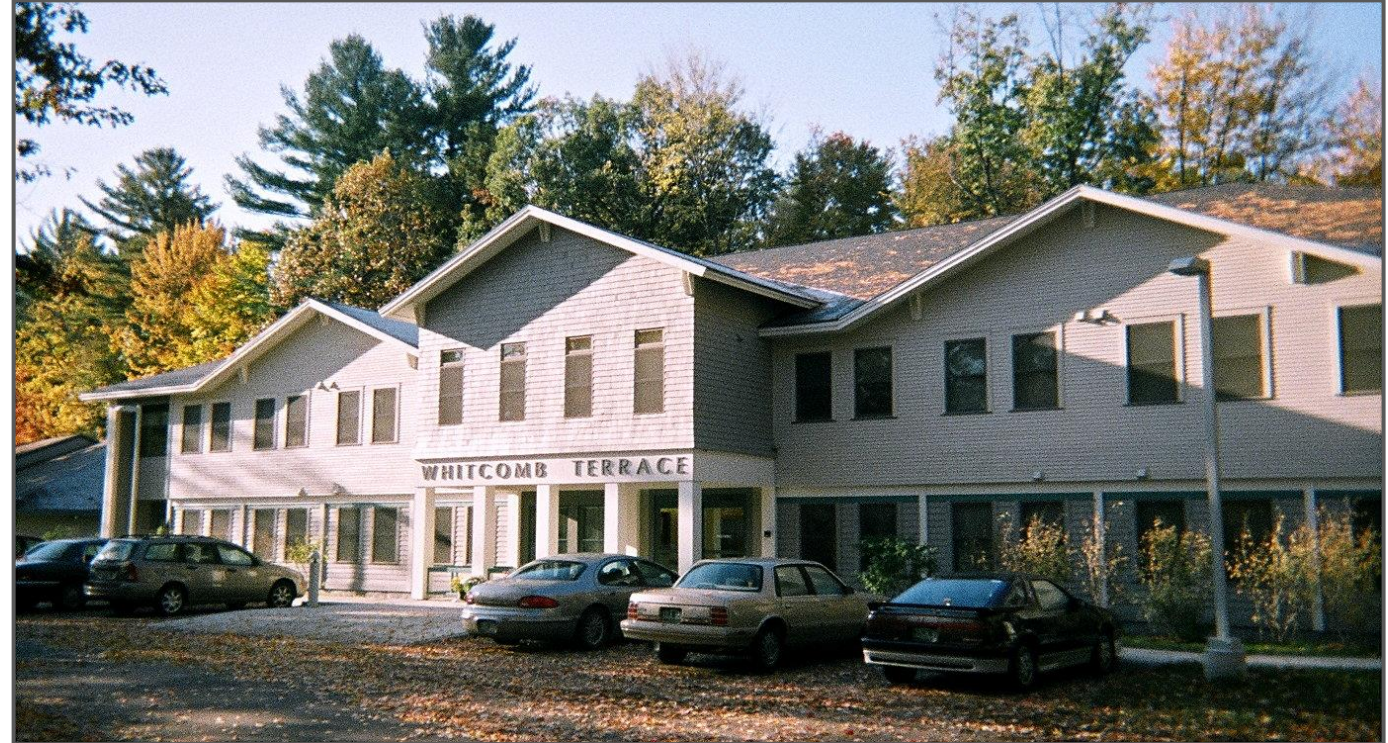
Whitcomb Terrace, 19 new units constructed on same site in 2004
