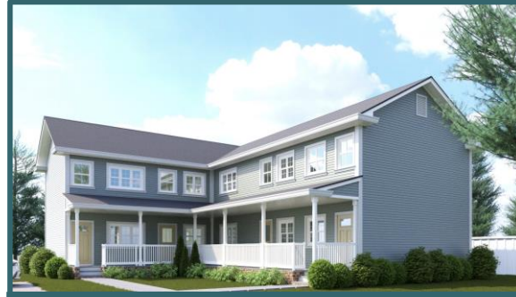
Bridge + Main A 19-unit, $7.2m scattered site affordable housing project currently in pre-development.
