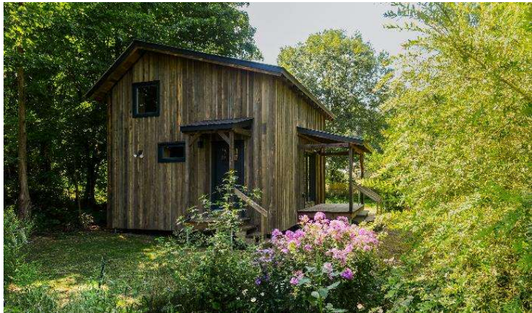
New Frameworks panelized 900 SF ADU with compressed straw bale exterior walls
