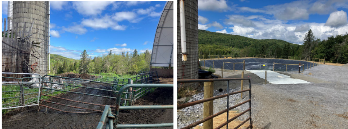
Figure 2. (Left) Before the project, this access road was utilized to move manure to an uncollected stacking location. (Right) After, in the same location there is a new greywater runoff collection system and the installation of a gravel mortality stack pad.
