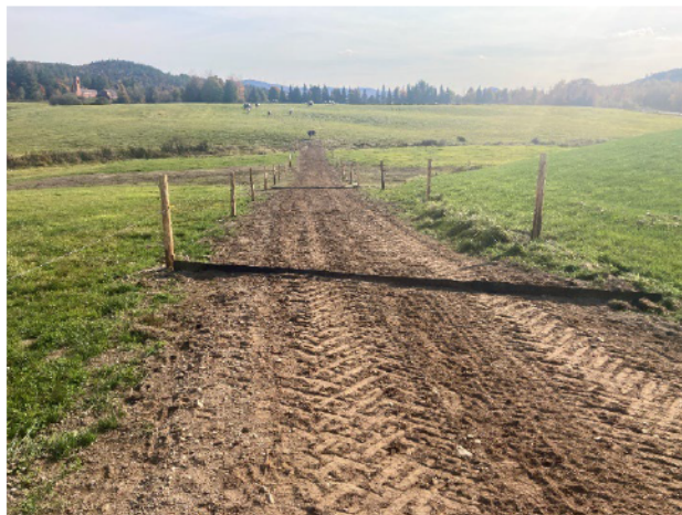
Figure 7. (Left) Animal trail installed to support movement into pastures with reduced impacts on water quality. (Right) Dairy cows rotationally grazing in pastures on Spring Brook Farm.
