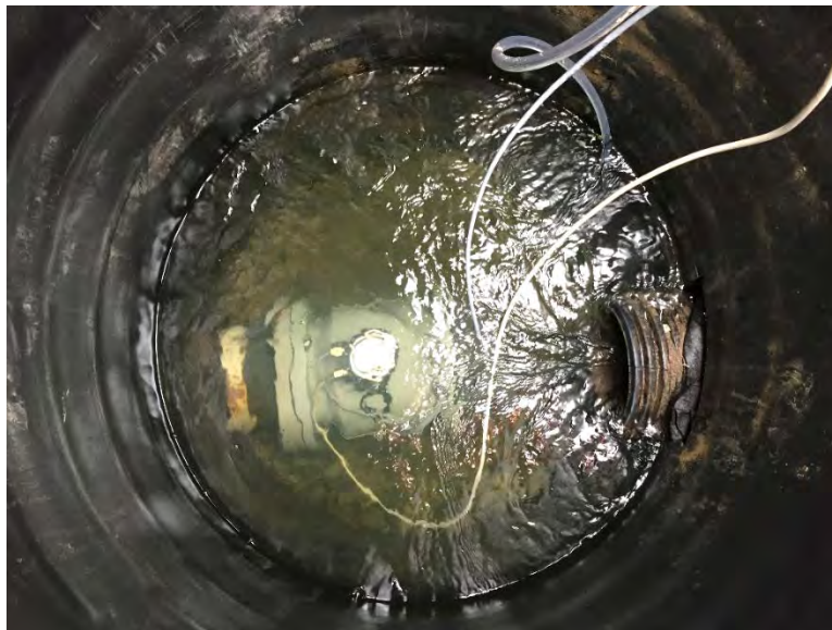
Figure 7. 8-inch Waterflux 3000 flowmeter in JBT11 manhole
