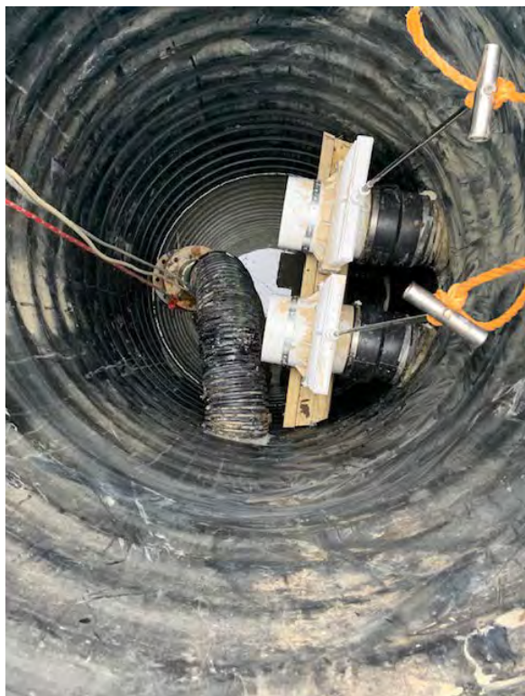
Figure 14. View down filter outlet manhole
