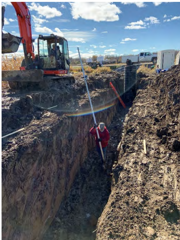
Figure 12. Excavating trench for Filter B
