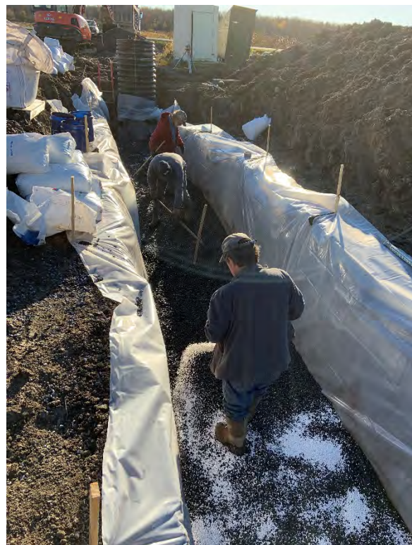
Figure 13. Spreading and raking in activated alumina and iron
