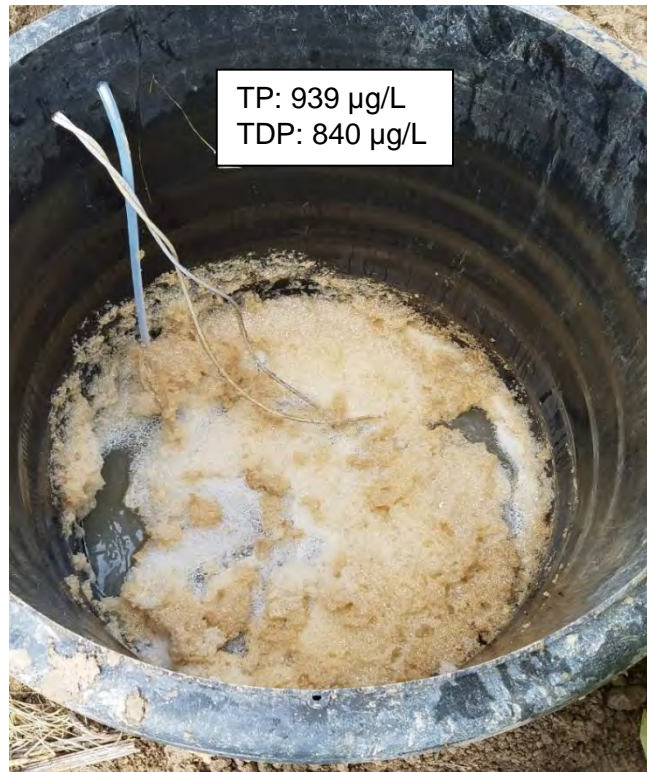
Figure 24. Foam in ACT4 manhole, Dec. 3, 2018
