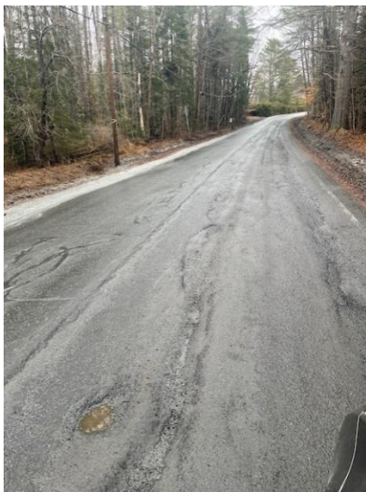
Marshfield Road, reclamation/repaving Planned for FY27
