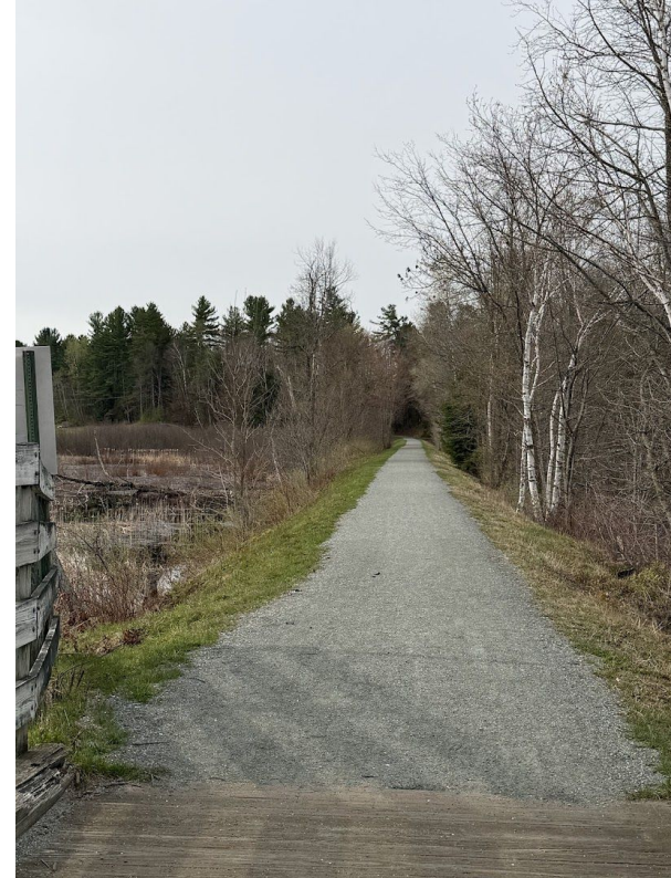
7' path into 8' wide trestle
