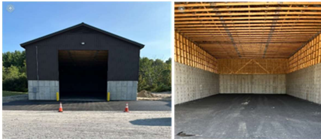
2024 - New Haven and North Hero Salt Sheds Completed
