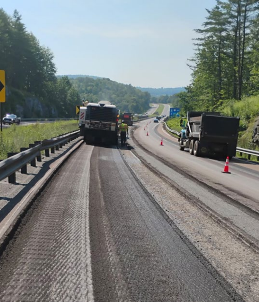
Milling the Passing Lane, Main Line
