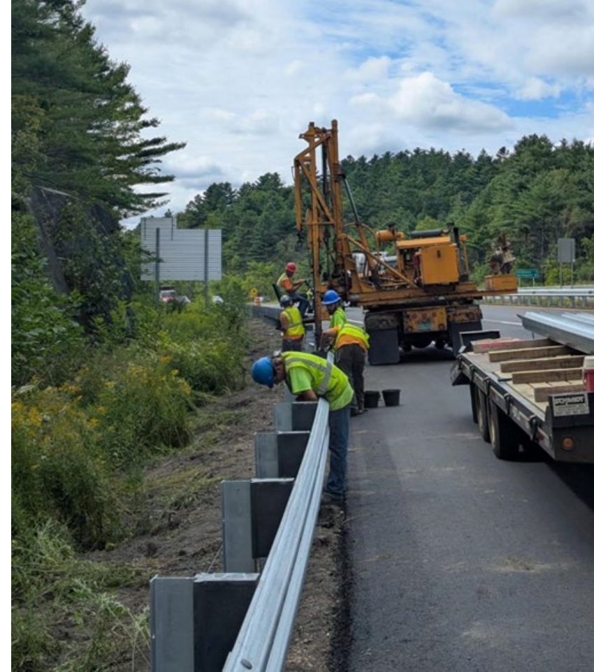
Installing New Guardrail
