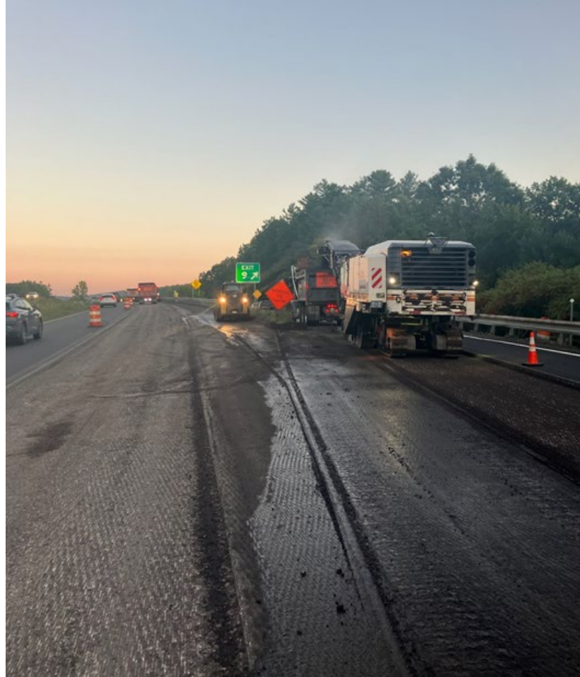
Milling Exit 9 Off Ramp
