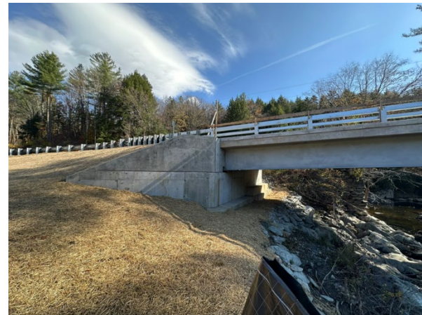
Worcester Bridge 84 on VT 12 After
