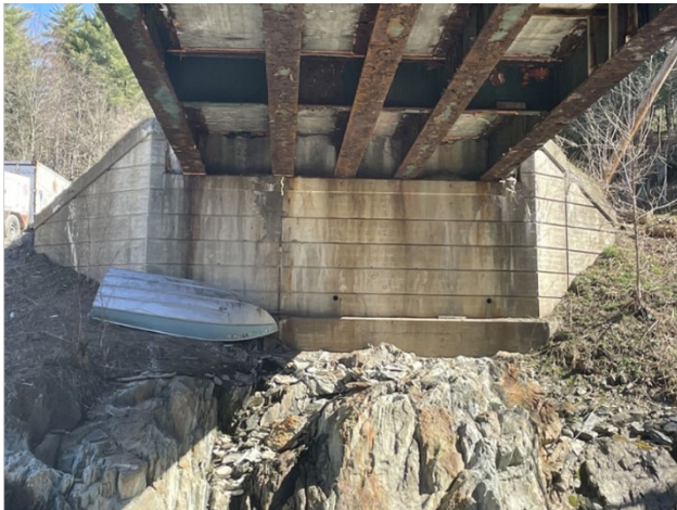
Worcester Bridge 84 on VT 12 Before
