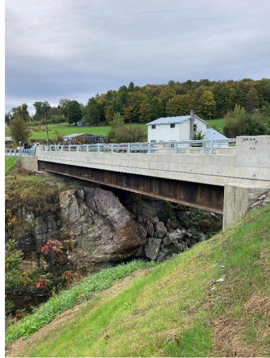
Fairfield Bridge 6 on VT 36 After
