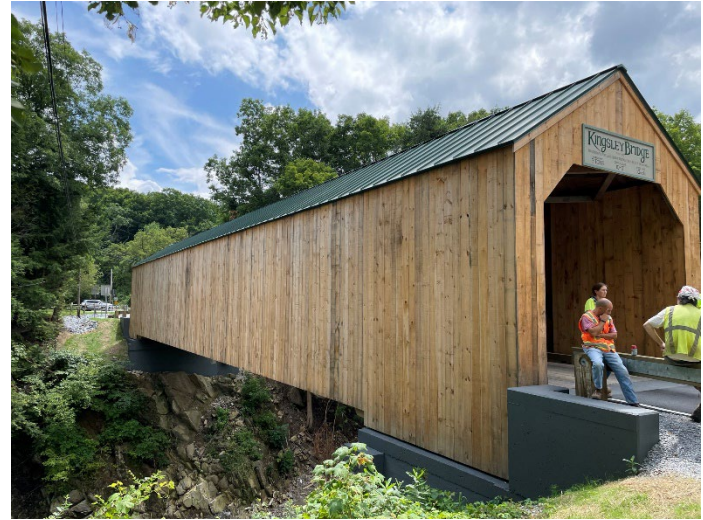
Kingsbury Covered Bridge on TH 39 in Clarendon After
