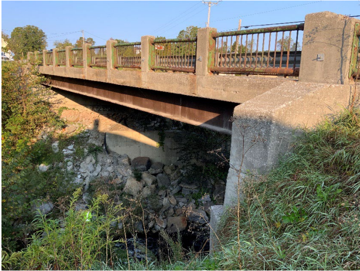
Fairfield Bridge 6 on VT 36 Before
