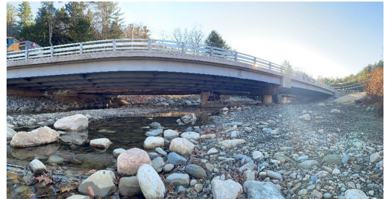
Grafton Bridge 20 on VT 121 After
