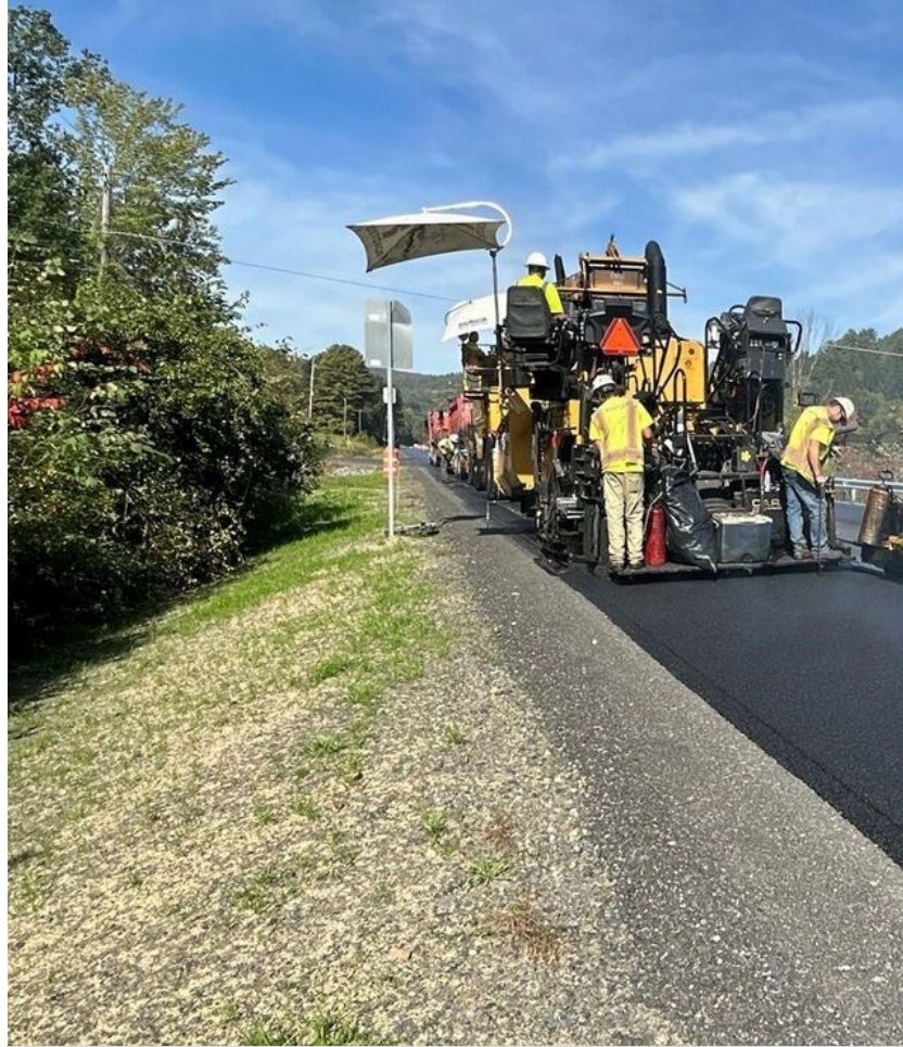
Paving with New Hot Mix
