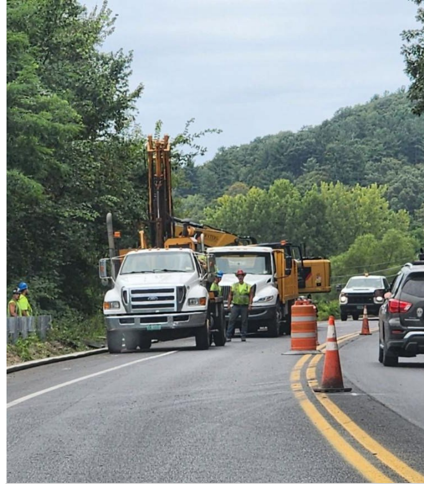
Installing New Guardrail
