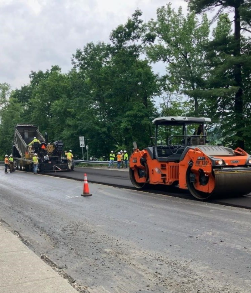
Paving with Plant Mix (Recycled Asphalt Pavement)
