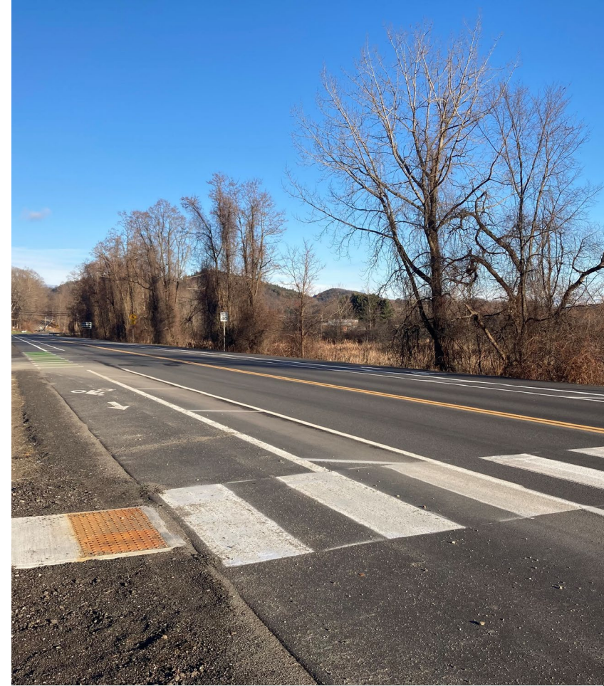
Installing New Crosswalk and RRFB
