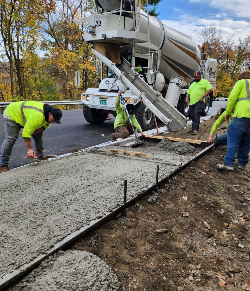
Rebuilding Sidewalk from Construction Impact
