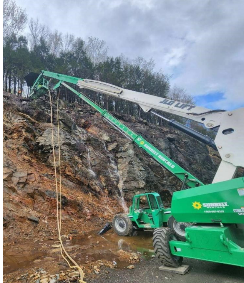
Rock Slope Scaling and Stabilization
