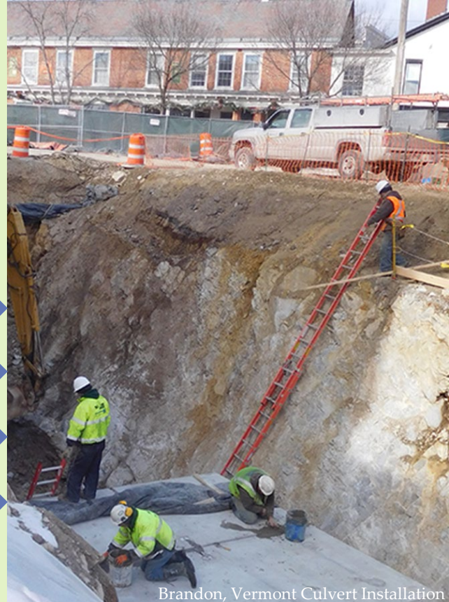
Brandon, Vermont Culvert Installation
