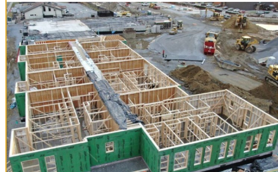
Bay Ridge, Shelburne Photo credit: DEW Construction
