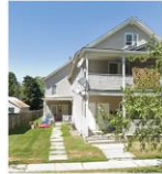
Main St, Essex Junction VT
