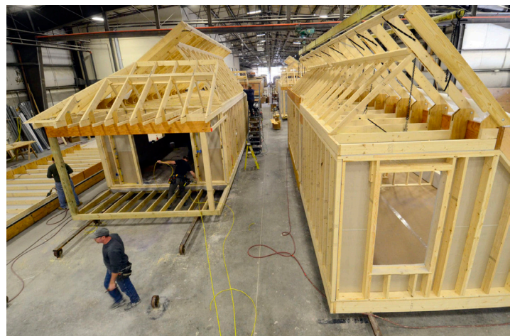
Off-site construction such as panelized (top) and volumetric modular (bottom) can dramatically increase the speed of housing production in Vermont. Credit: Bensonwood (top) and Huntington Homes (bottom)
