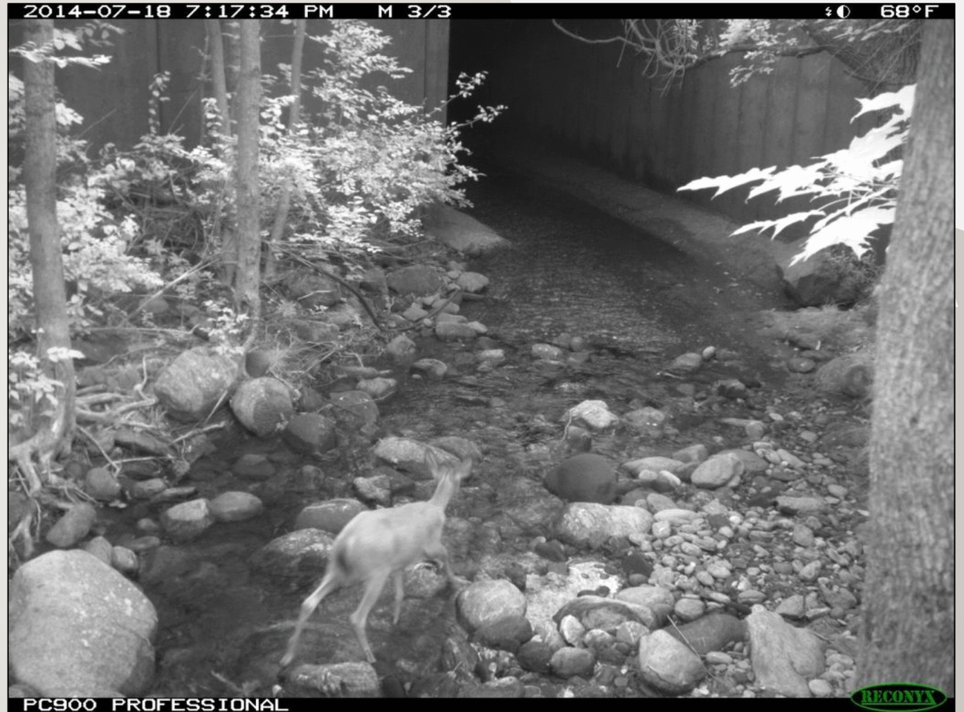
Pinneo Brook Culvert
