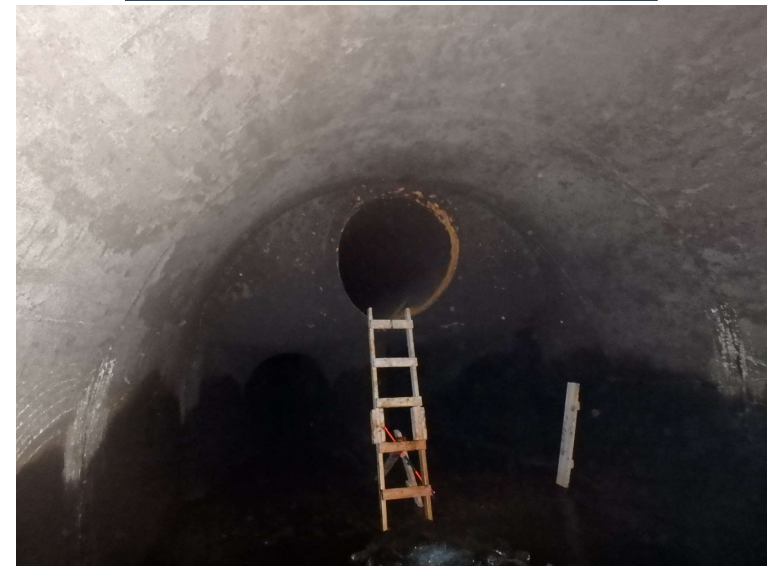
Waterbury Dam Tunnel
