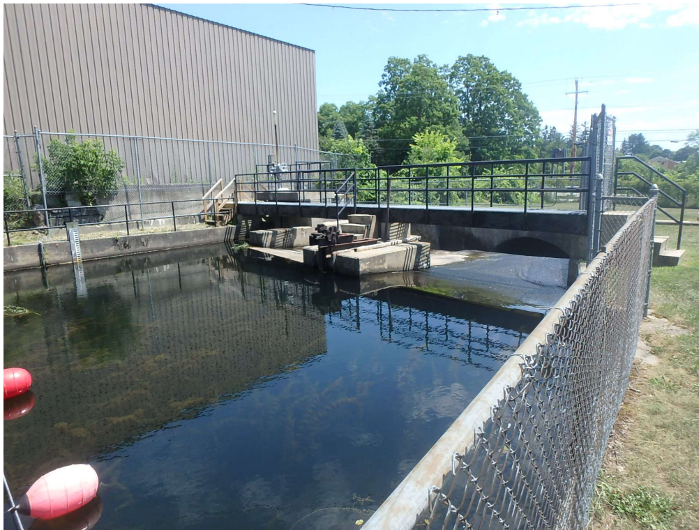
Lake Bomoseen Dam, Castleton
