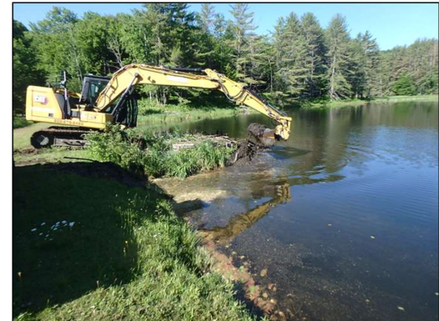
CCC Pond Dam, Addison
