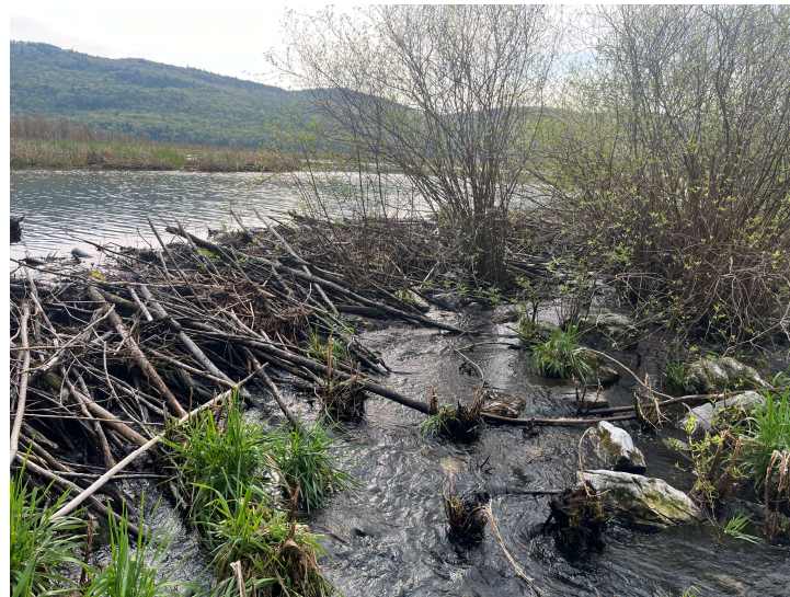
Lake Winona Dam/Bristol Pond Dam, Bristol
