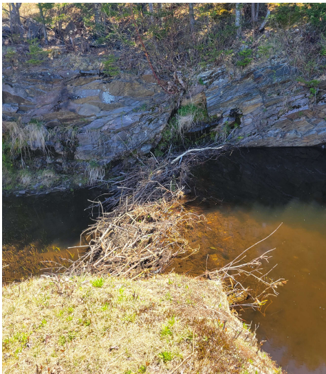
Wolcott Pond Dam, Wolcott
