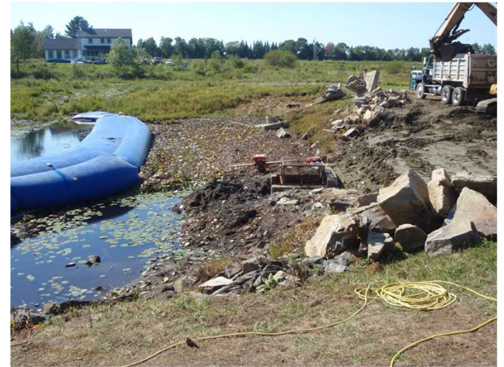
Wolcott Dam Rehabilitation, Vermont, 2015
