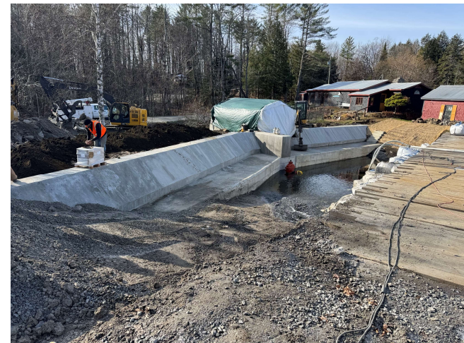
Curtis Pond Dam Rehabilitation, Calais
