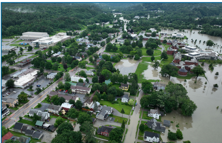
Flooding in Waterbury, VT 2023. Since 2011, the Lake Champlain Basin has been impacted by all 22 major FEMA declared extreme weather disasters in Vermont including three severe storms and flooding in 2023 and two in 2024.
