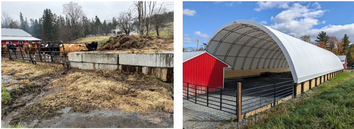
Figure 2. (Left) Uncovered barnyard had runoff issues in wet conditions. (Right) New covered barnyard area provides a clean area for manure storage and livestock and eliminates runoff concerns.
