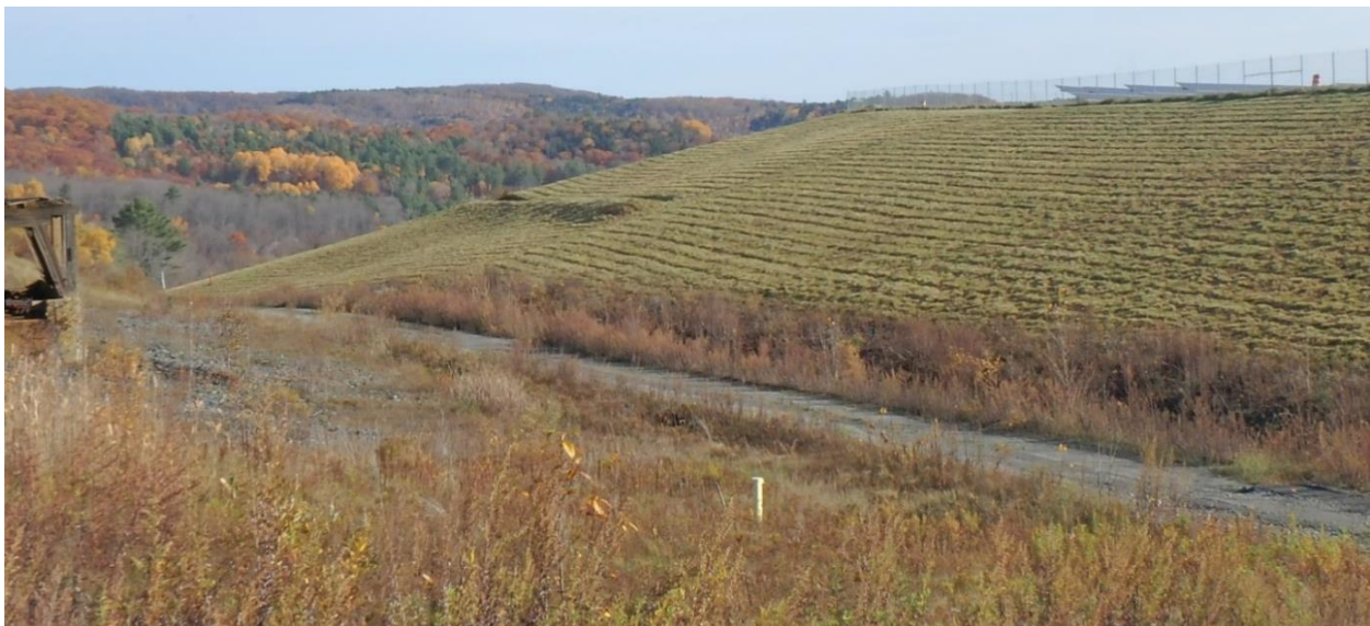
Elizabeth Mine Tailing Pile 1 Dam in Strafford – A HIGH Hazard Potential Dam Impounding mine tailings and contaminated groundwater and surface runoff which is treated before being discharged to Copperas Brook
