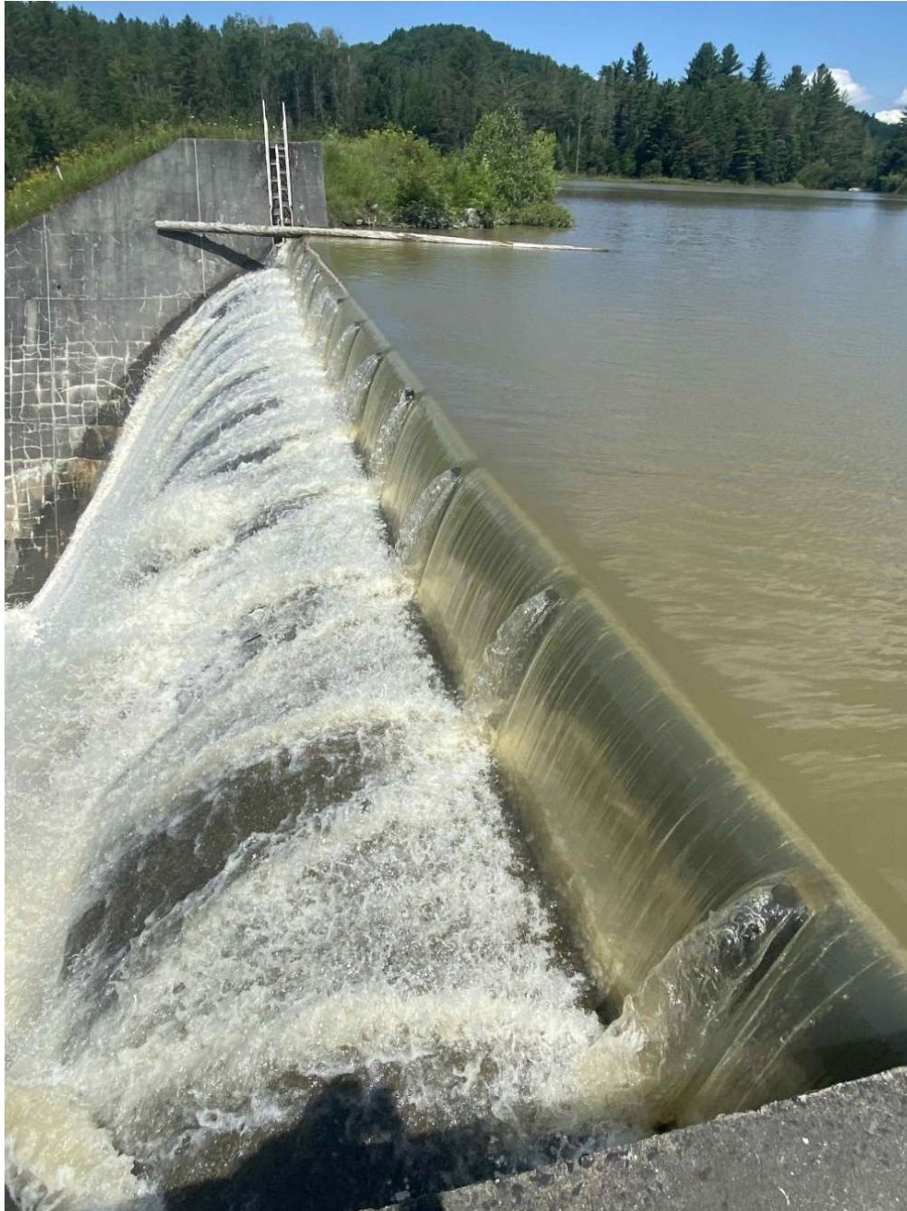
Overflowing Spillway Chute at Thurman Dix Reservoir Dam in Orange in July 2024 This municipally owned HIGH Hazard Potential Dam impounds the City of Barre’s water supply
