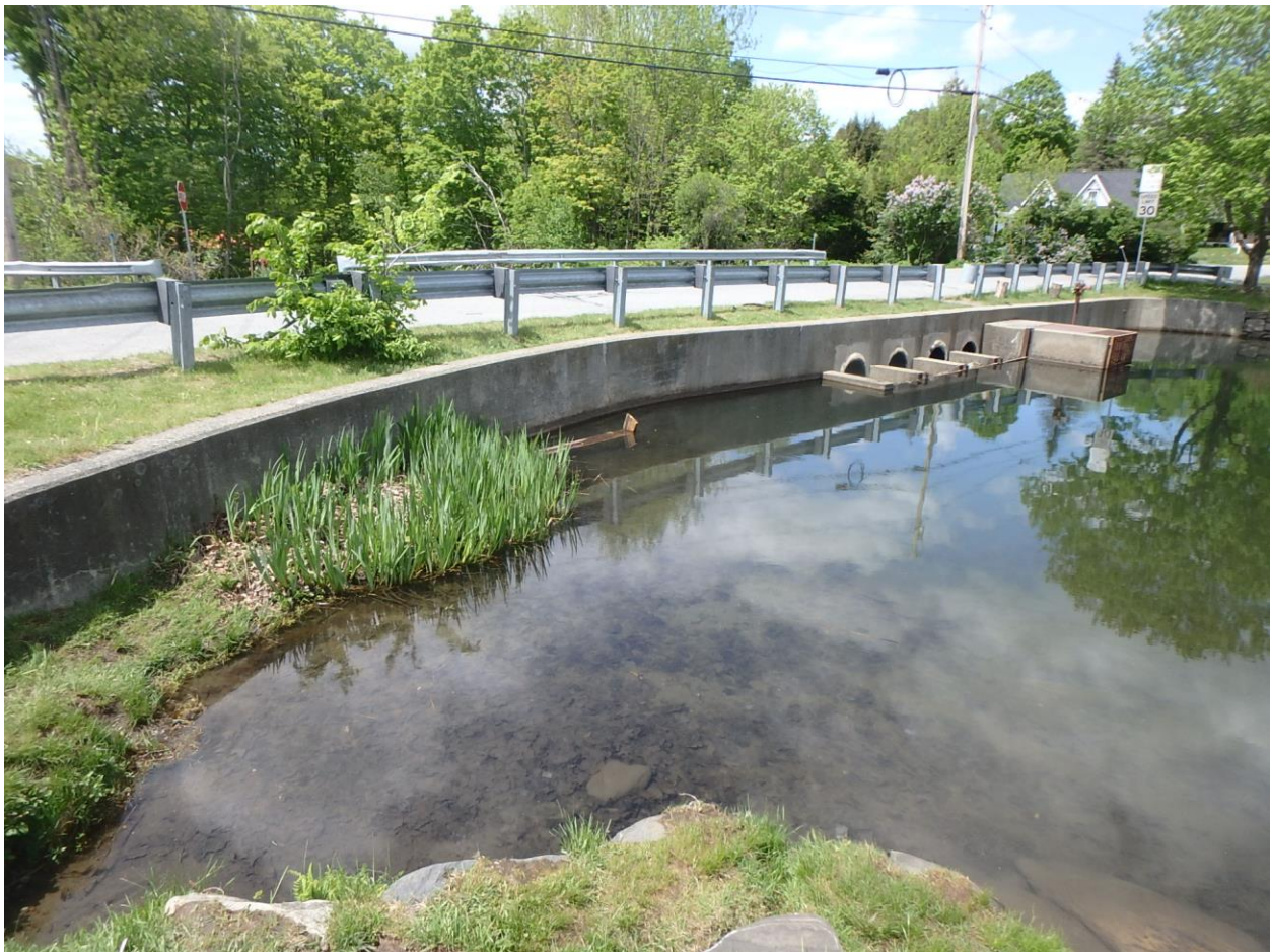
Silver Lake Dam - This State-owned HIGH Hazard Potential Dam has a roadway on the crest of the dam
