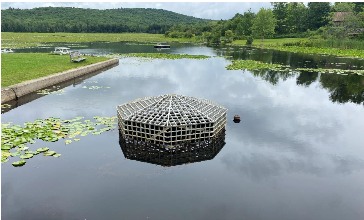
The Spillway Riser at Municipally Owned Star Lake Dam in Mount Holly
