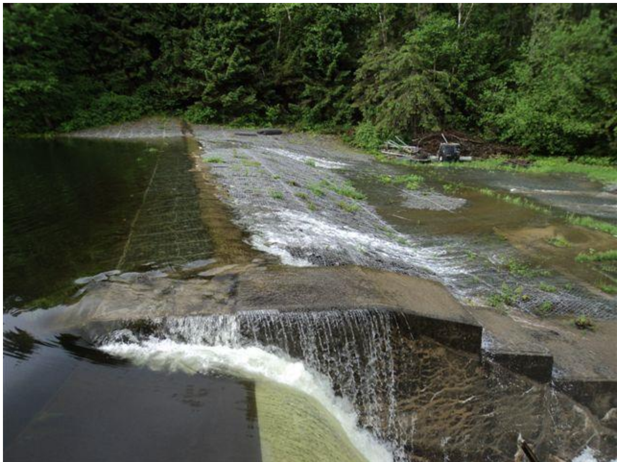
Spring 2011 Overtopping of Stiles Pond Dam, a Municipally Owned HIGH Hazard Potential Dam in Waterford
