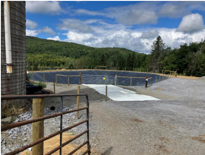
Figure 17: A new greywater collection pit installed on a small dairy farm operation in the Winooski river basin. The project included a bedded pack facility for winter livestock management, heavy use area improvements, and a covered manure stacking area. This small family dairy farm previously managed their farm with an outdated liquid storage tank and uncovered manure storage areas. This project was supported through the Best Management Practices (BMP) Program in collaboration with federal partners.
