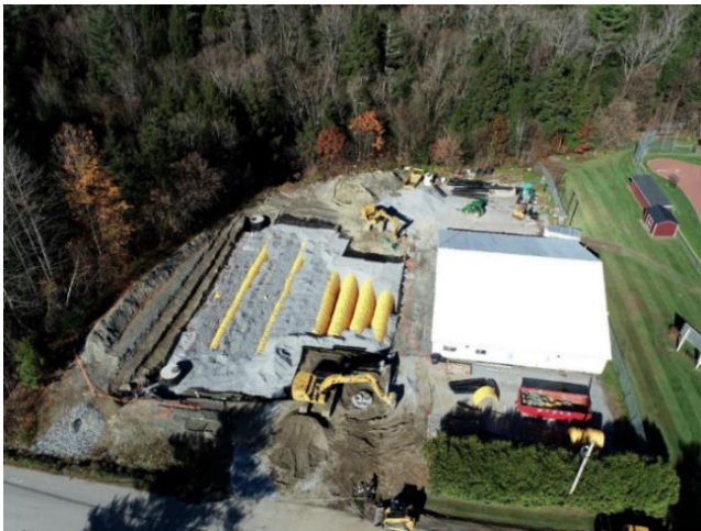
During construction photo of a subsurface sand filter system constructed at Bellows Free Academy in Fairfax, VT as part of the Green Schools initiative.
