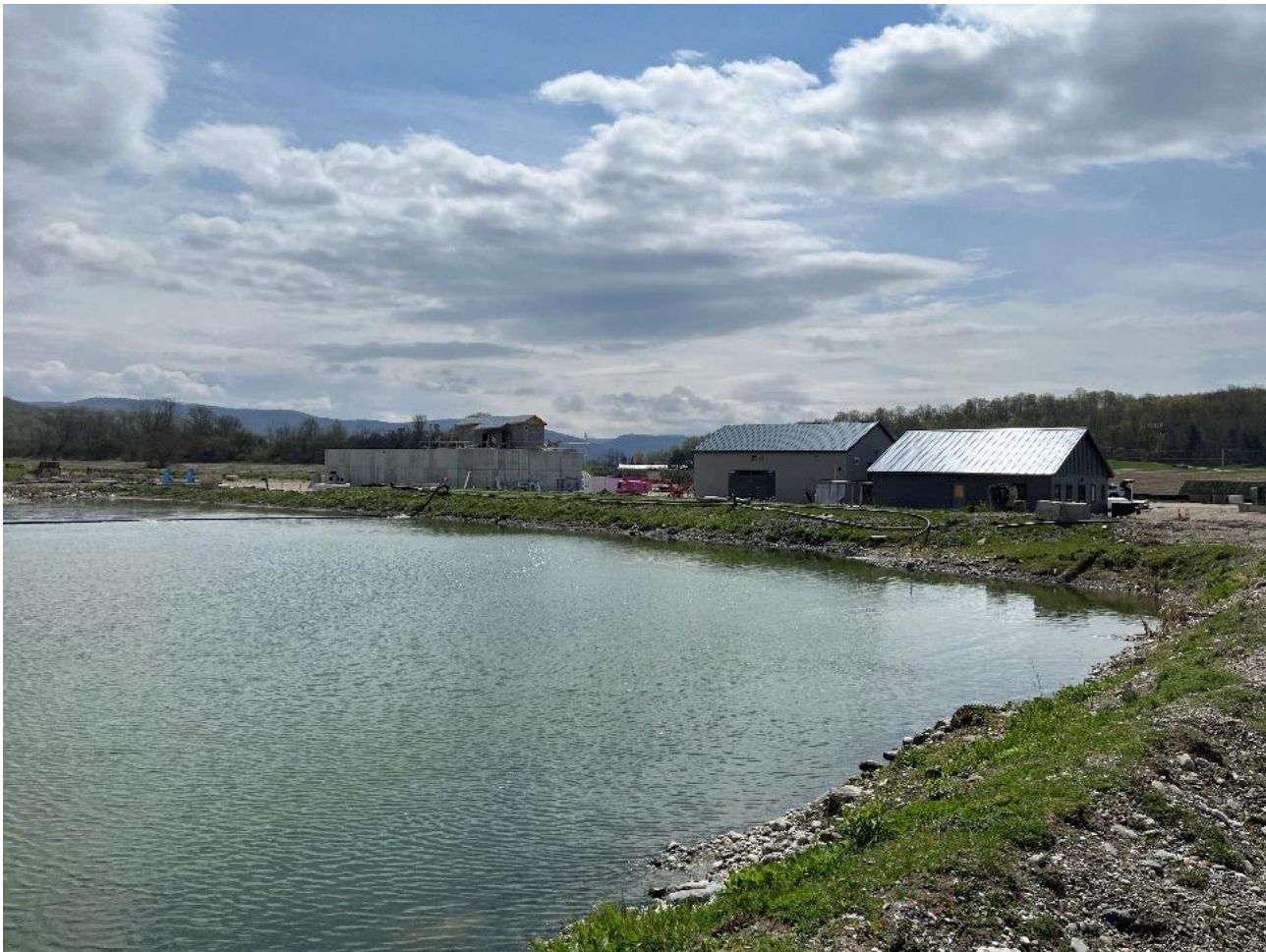
Figure 19: Town of Hinesburg wastewater treatment facility under construction, with existing lagoon in the foreground. Hinesburg is upgrading to better treatment technology to treat for phosphorus removal as part of the Lake Champlain TMDL, nitrogen removal as part of a local ammonia water quality issue, and a small increase in hydraulic capacity to be able to add housing and new users. A future phase of the project involves floodplain restoration. The town of Hinesburg has partnered with the State of Vermont to finance this project in part by low-interest loans available through the Clean Water State Revolving Fund.
