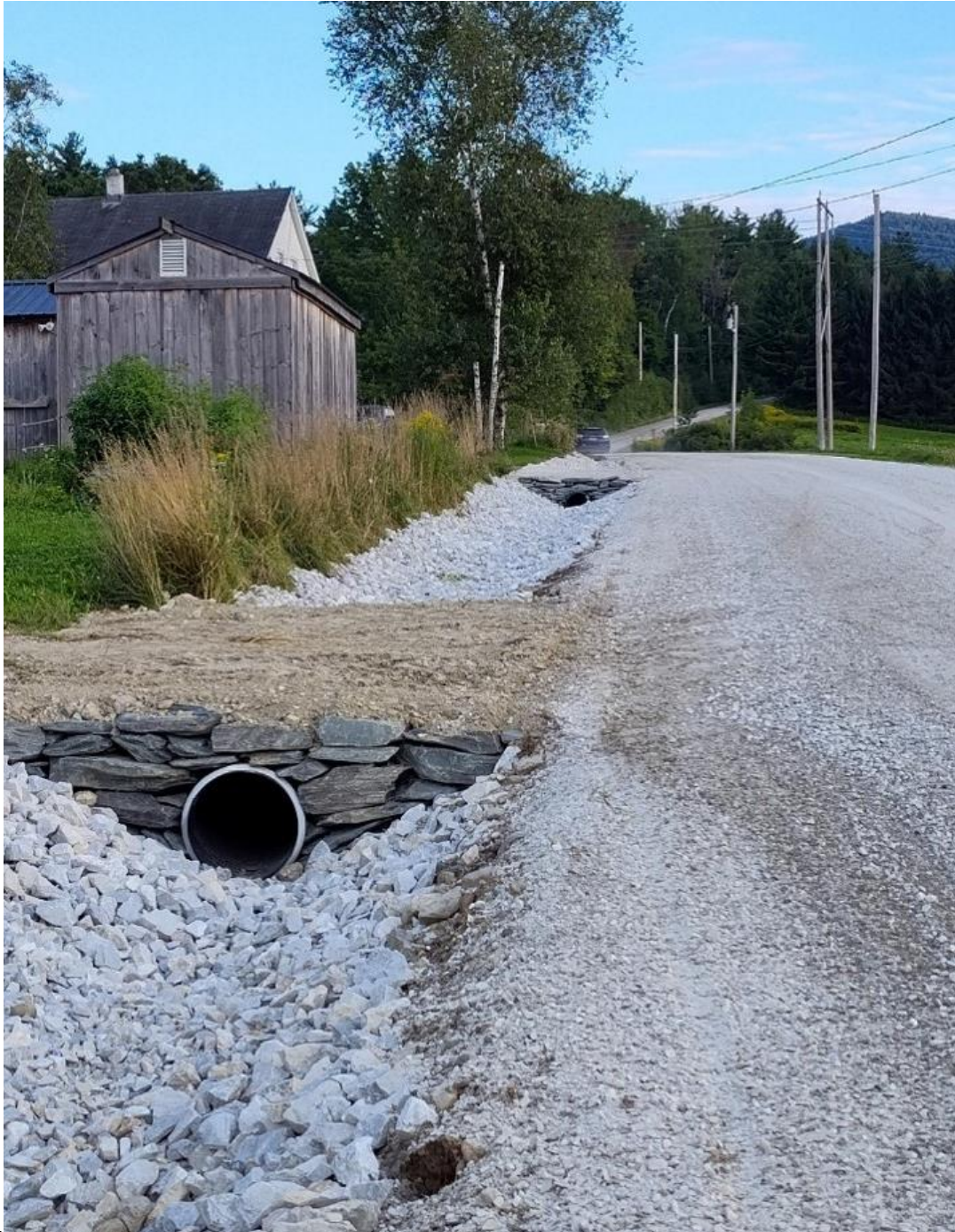
Figure 19: Stormwater erosion control improvements on Birdseye Road in Ira, VT. Best management practices (BMP) like this are implemented in accordance with the Vermont Department of Environmental Conservation's (DEC) Municipal Roads General Permit (MRGP) on eligible road segments that are not fully compliant with MRGP standards. Project work was funded by the VTrans Grants-in-Aid Program (coordinated by Dan Judkins, VTrans Grant Coordinator) and implemented by the VTrans Better Roads Program (coordinated by Ross Gouin, VTrans Better Roads Program Manager). Road improvements like these reduce sedimentation into Vermont's surface waters. This project was completed in August 2025.
