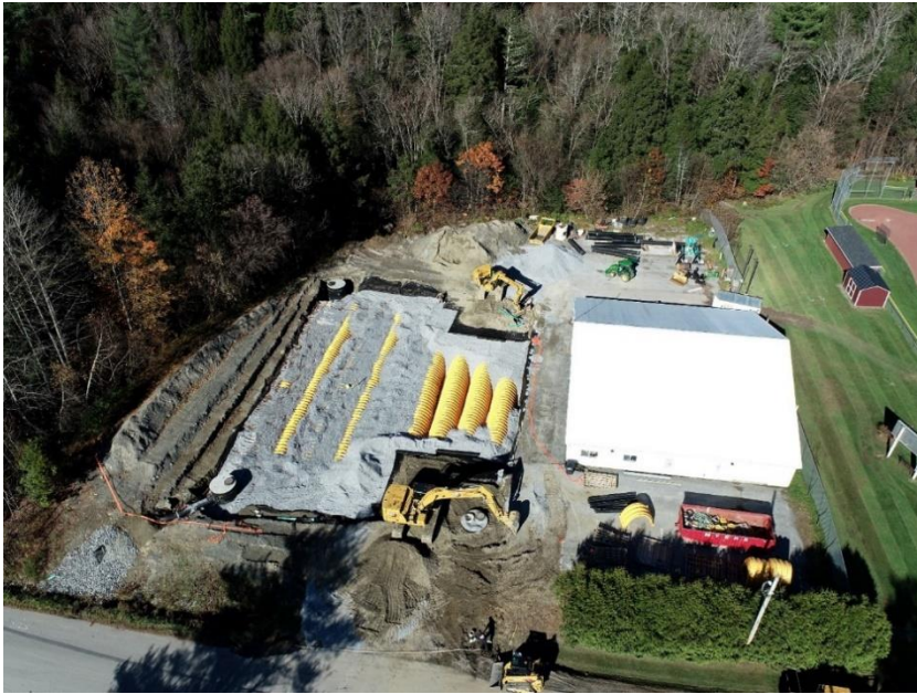
Figure 20: During implementation photo of a subsurface sand filter system constructed at Bellows Free Academy in Fairfax, VT as part of the Green Schools initiative. Sand filter systems remove pollutants from stormwater runoff by allowing heavy solids to settle out, after which stormwater passes through a layer of sand and gravel, removing smaller particles. This project was funded through a DEC-program with Lake Champlain Basin Program (LCBP) and American Rescue
