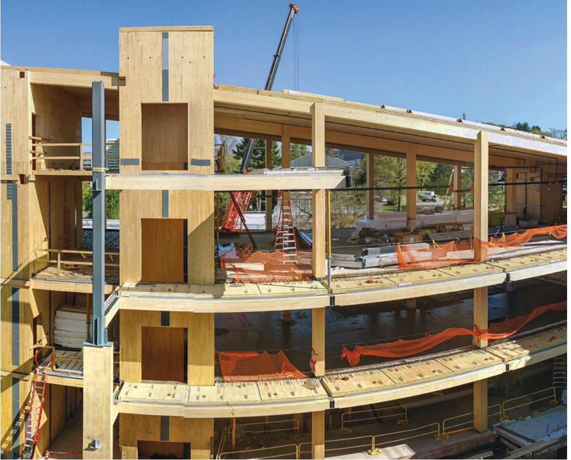
The John W. Olver Design Building at the University of Massachusetts Amherst has a unique cross-laminated timber structural system, which reduces its carbon footprint.
