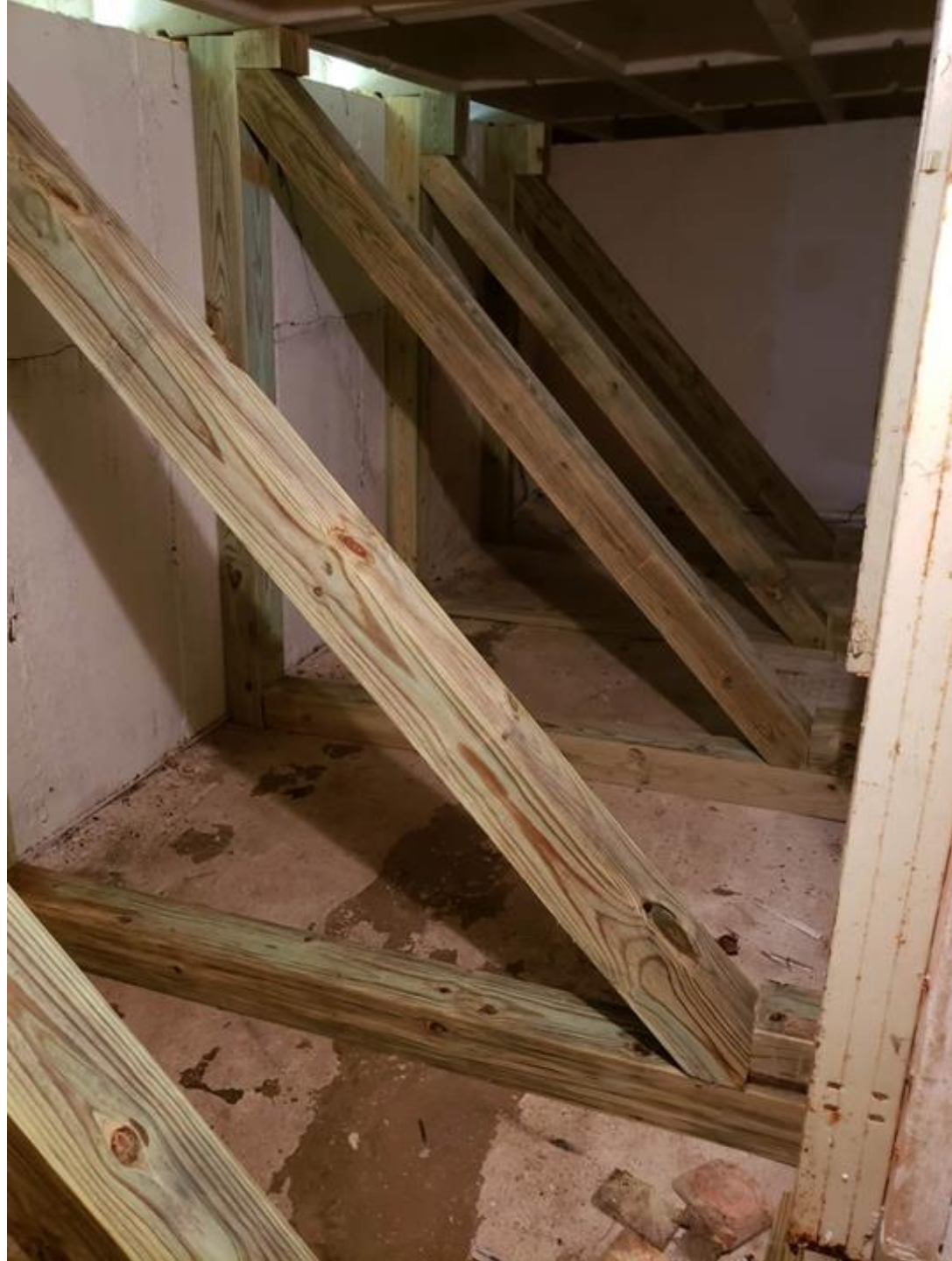
West wall bracing
