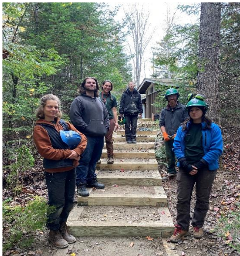
A proud VYCC crew poses with their completed timber stairs at Stillwater State Park campground.
