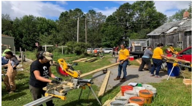
Hartford Trailblazers building an accessibility ramp for a community member.
