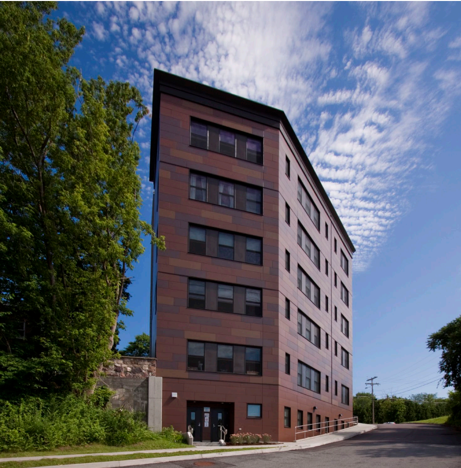
Canal Street Veteran Housing, Winooski
