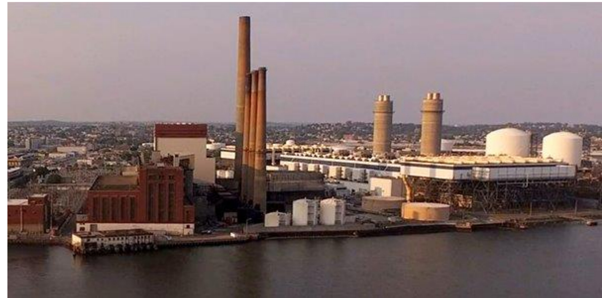
Mystic Generating Station in Everett, MA
