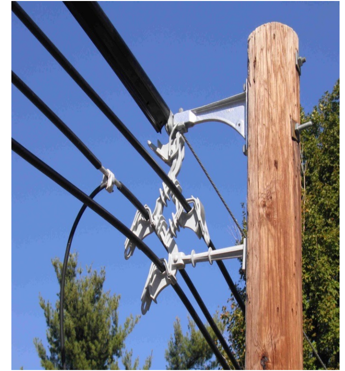
Spacer Cable-Steel Messenger Reinforced Covered Wire
