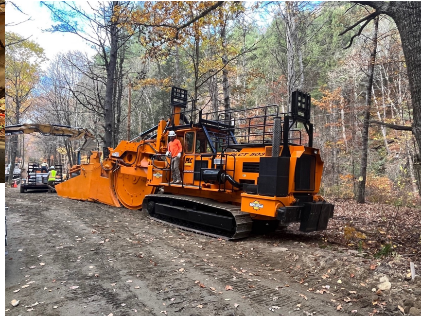
Underground Installation- Rock Saw
