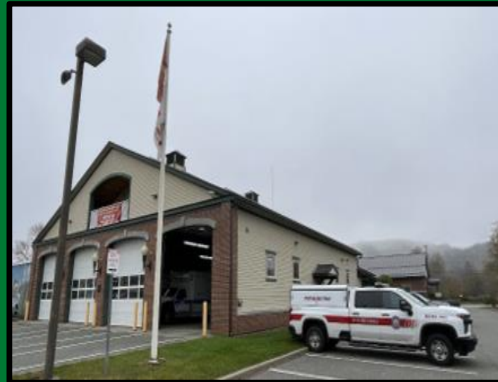
Lyndon Public Safety Building
