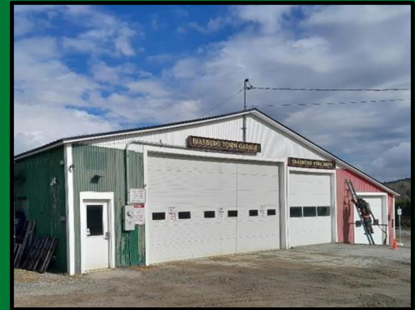
Irasburg Town Garage and Fire Station
