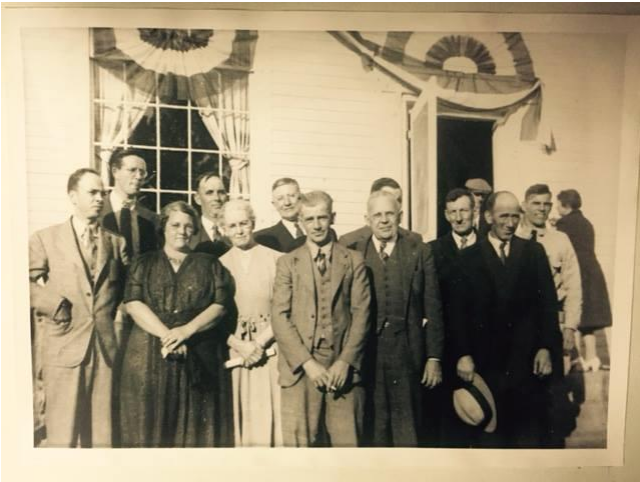
VEC Energization Day 1938
