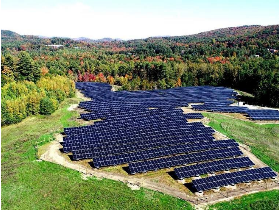
Photo courtesy of Encore Renewable Energy
