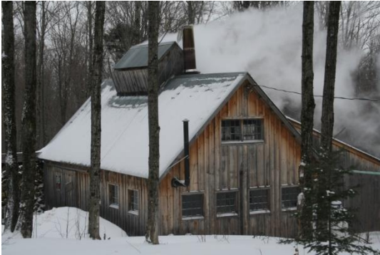
Little Charlie's Sugarbush (Jay): .57 mile line extension to displace 7,907 gallons of propane per year.
