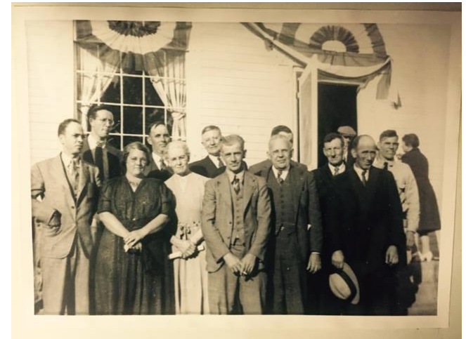
VEC Energization Day 1938
