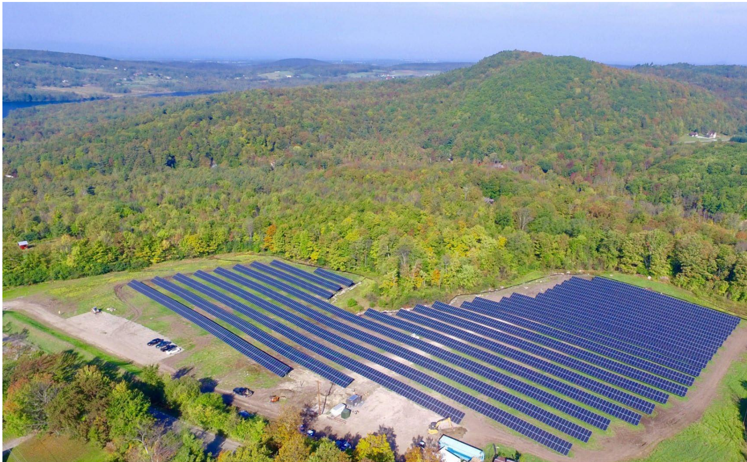
Photo: Courtesy of Encore Renewable Energy
