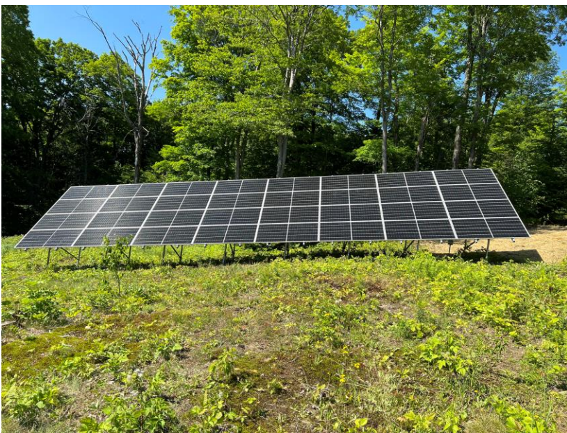
15kW residential solar array in Barnard
