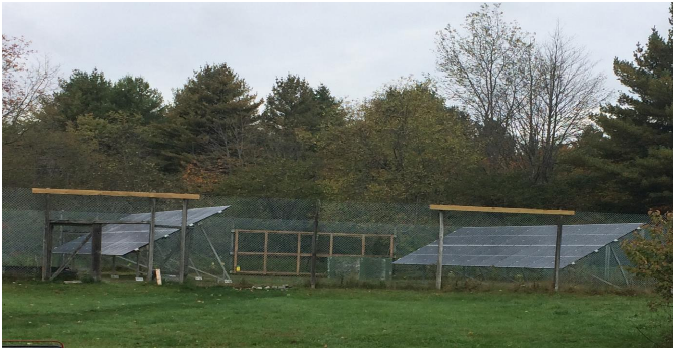
17kW Array in Southern Vermont
