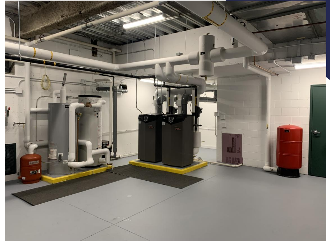
Franklin Elementary School, VT – 2022 - Oil to LP w/ Condensing Boilers
