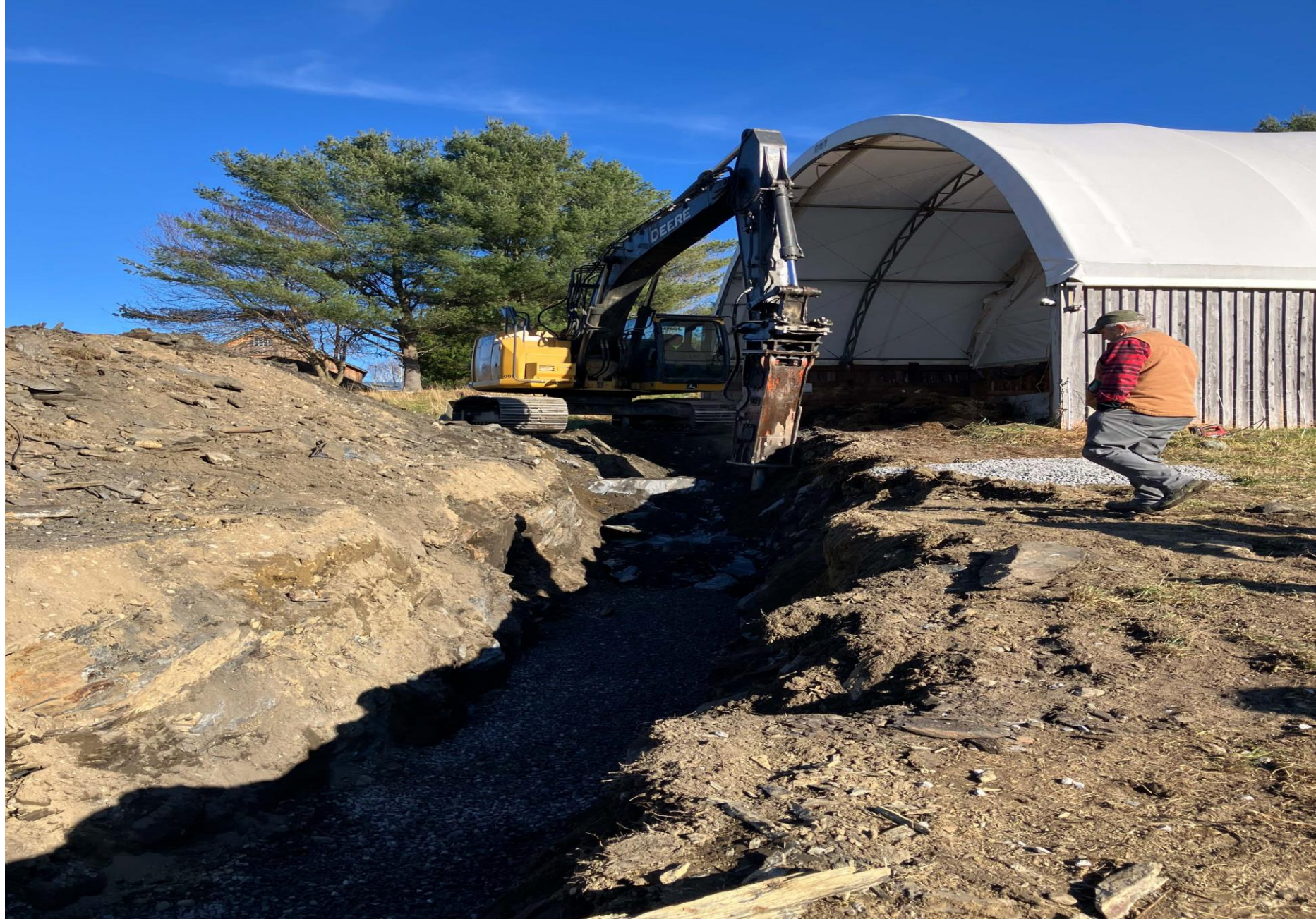
INSTALLATION OF WATER MAIN TO NEW SOURCE TO ADDRESS PFAS CONTAMINATION FOR CRAFTSBURY FD#2 WATER SYSTEM
